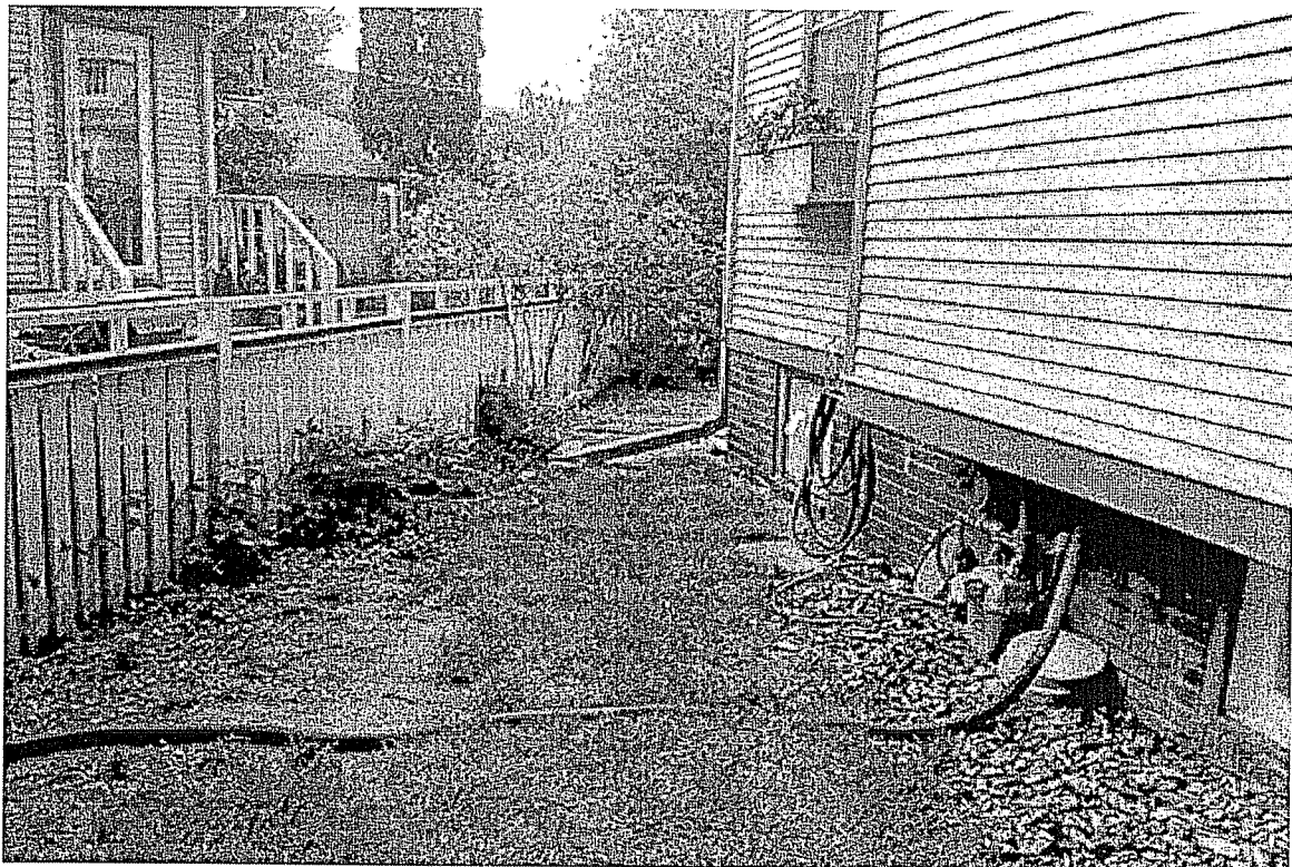
West side. Looking North to backyard.
