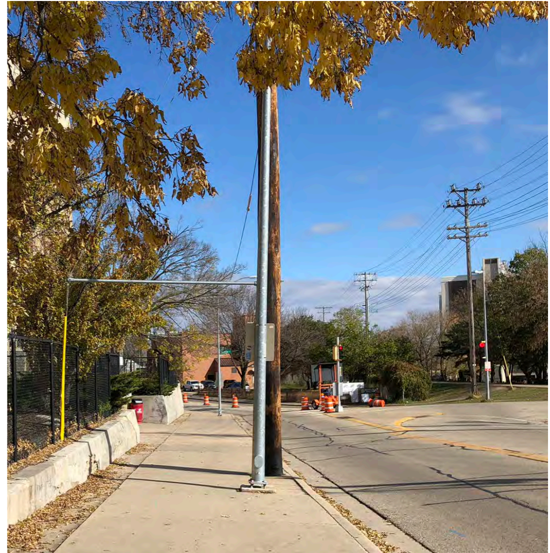
Utility Support Pole
