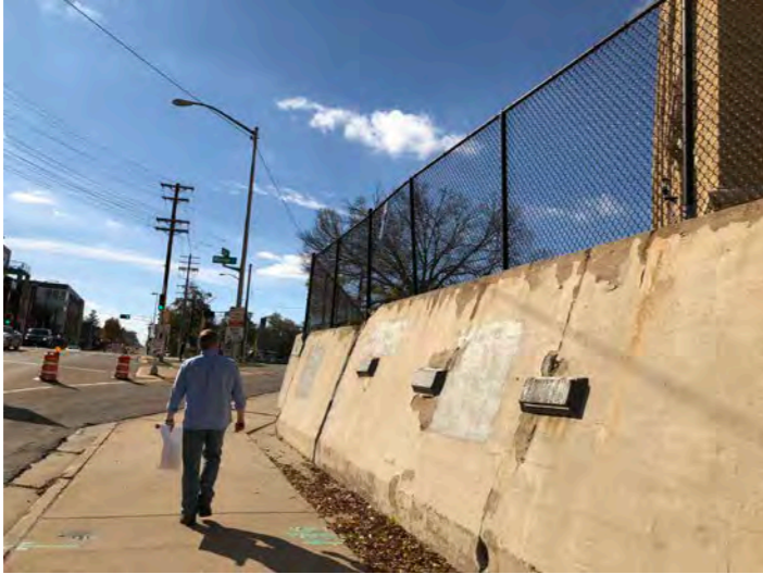
Existing Retaining wall
