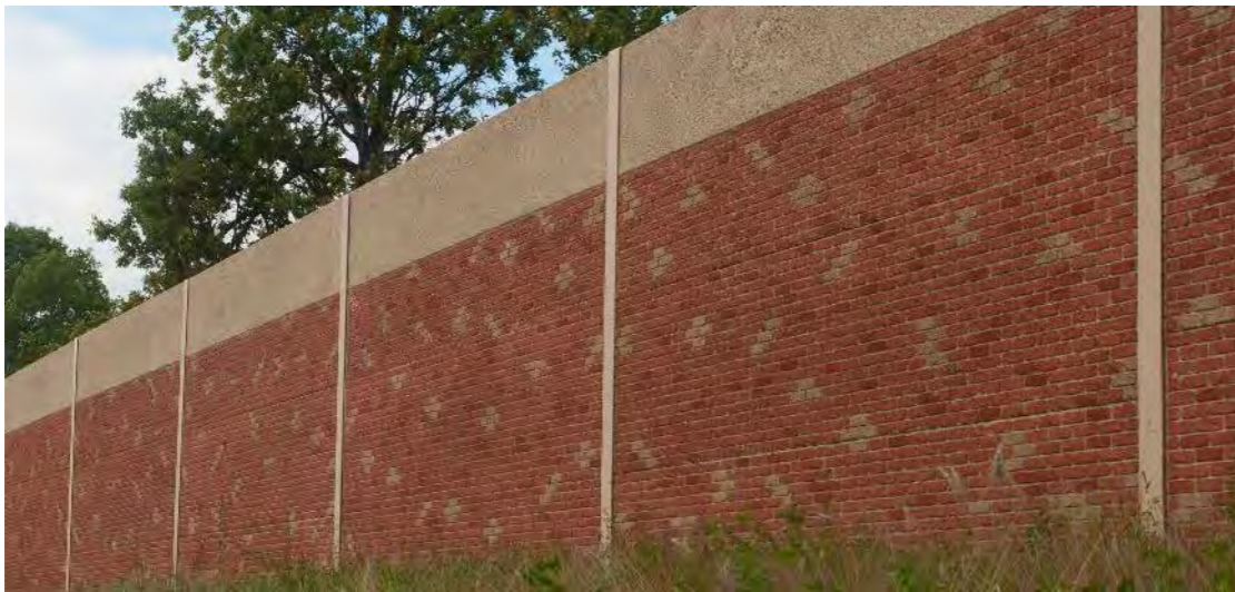
Brick Veneer Replacement Wall
