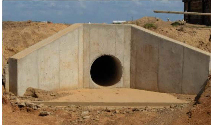
TYPICAL PIPE WITH NO SURFACE TREATMENTS
