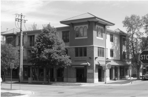
Figure D1: Entrance Orientation
