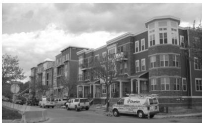
Figure D6: Building Alignment
