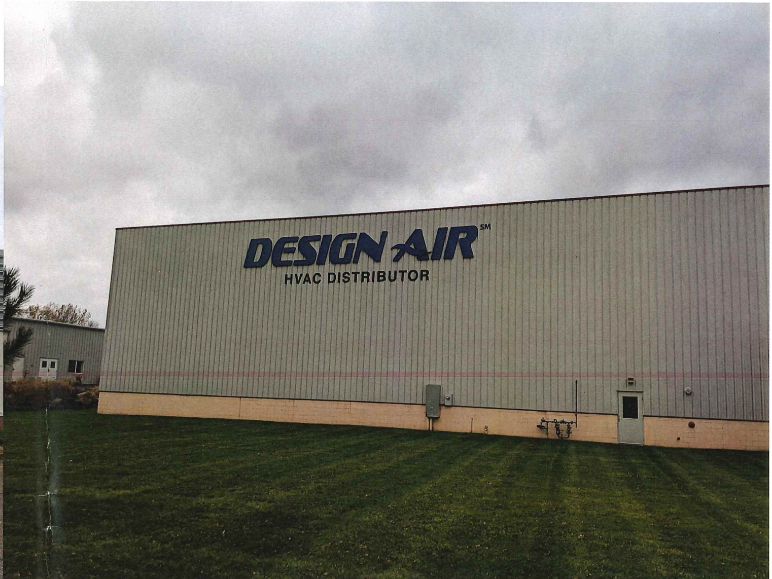
Design Air Located Immediately Northeast.
