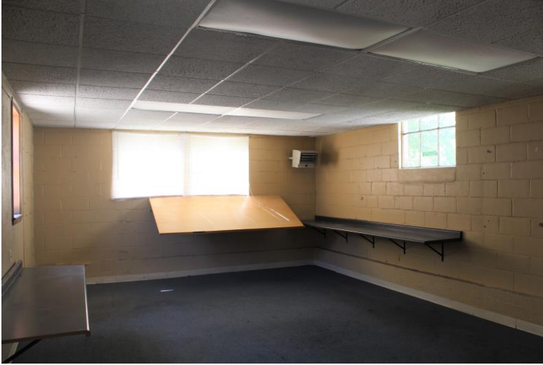
View of one of the work area/offices in the south addition.
