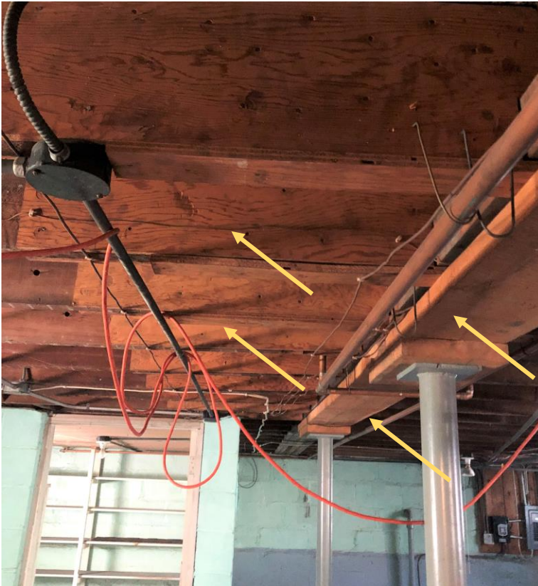
Modifications to floor joists and main beam in basement.
