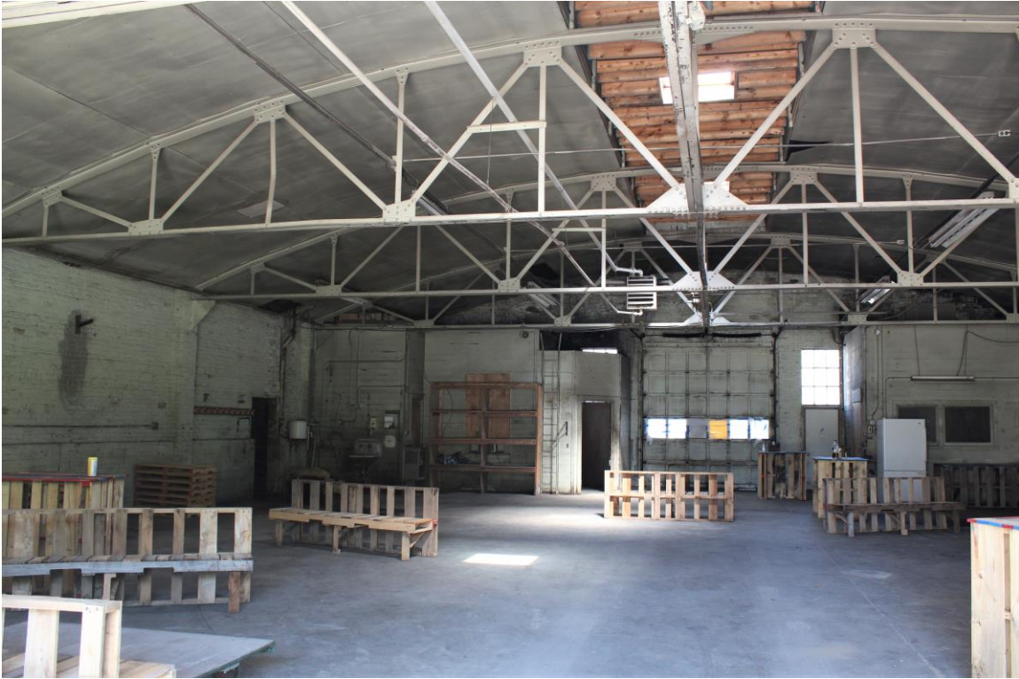
Interior of the original service garage looking north. June 20, 2022
