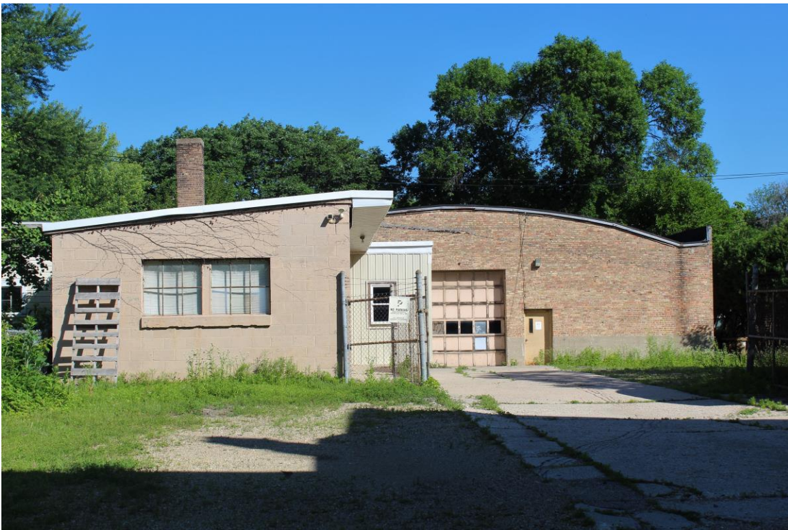
Rear view, 615 East Dayton Street. June 20, 2022
