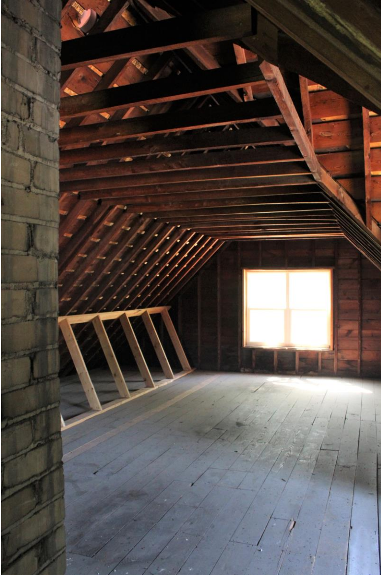
Unfinished attic looking toward Mifflin Street.
