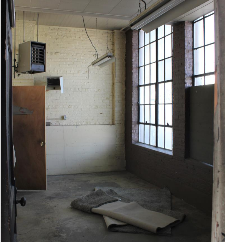
View of the office area within the original building. Note brick masonry walls and industrial steel windows.
