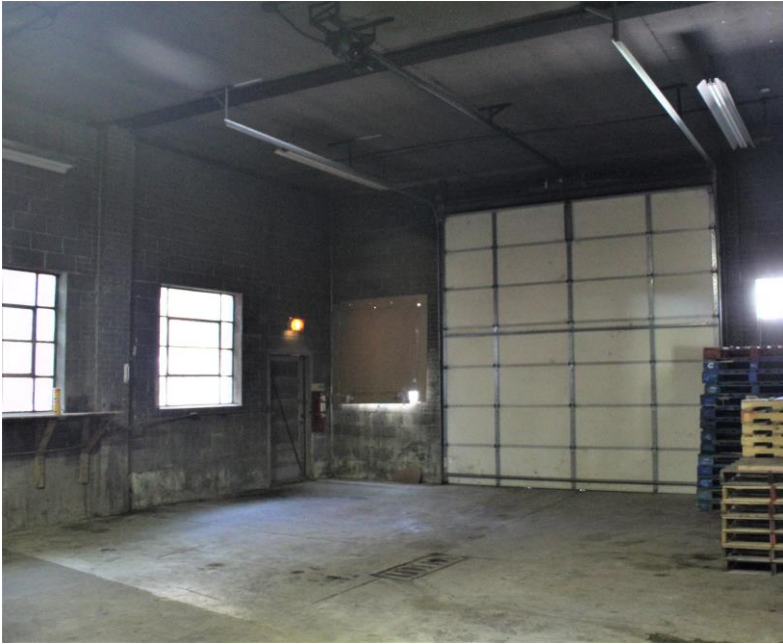
View of the interior of the west addition.
