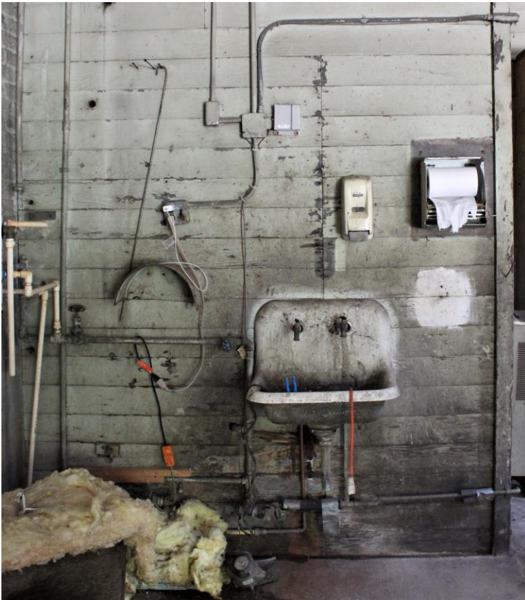
View of interior of main garage original building cleanup station.
