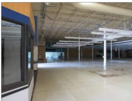
Former grocery store building is approximately 76,715 square feet.
