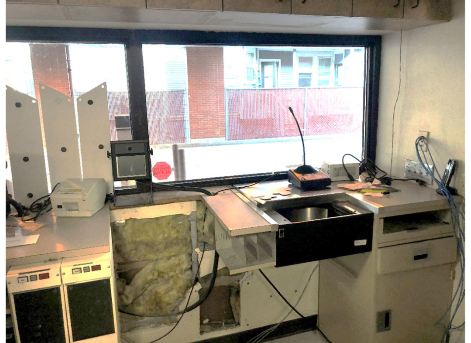
EXISTING INTERIOR, LOOKING TO VASSW AREA
