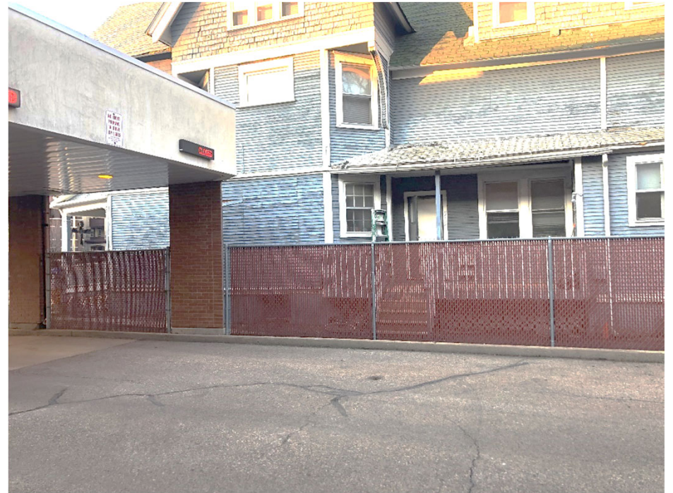
VIEW TOWARD NEIGHBORING RESIDENTIAL STRUCTURE
