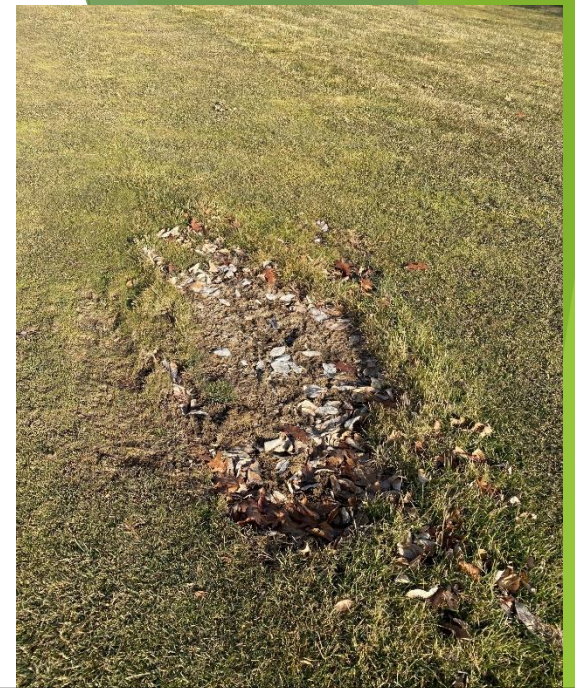
Monona irrigation head leak area visible in many areas of course.
