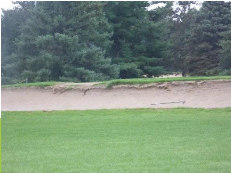
East #6 bunker collapse from overtime failure
