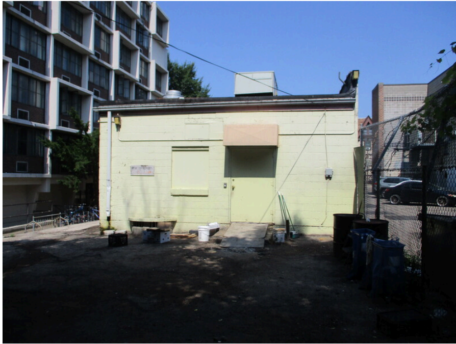
Photo 3: 411 W. Gilman Street-east side of building/property
