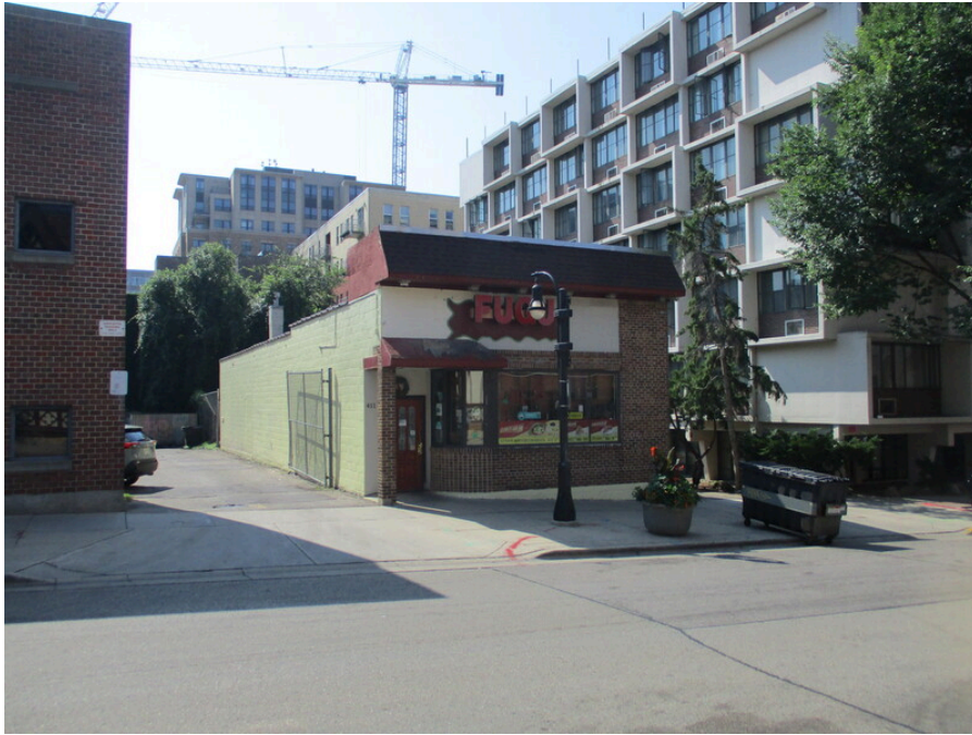
Photo 1: 411 W. Gilman Street-west and north side of building/property
