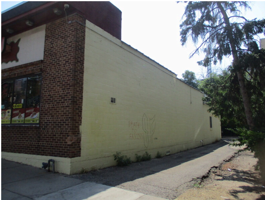
Photo 2: 411 W. Gilman Street-south side of building/property
