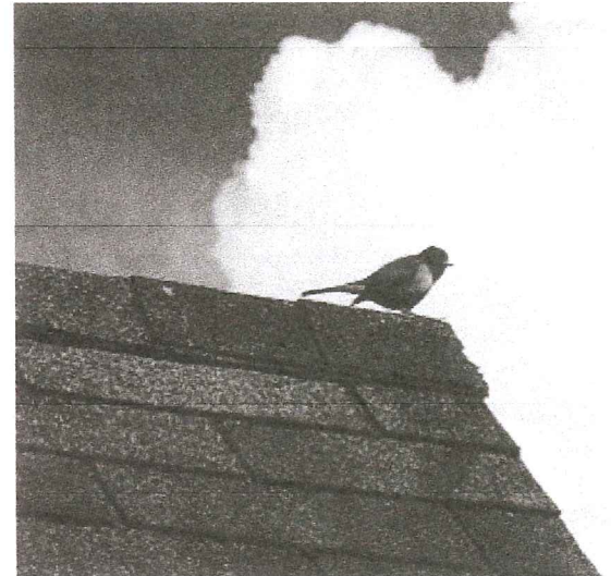
A ridge cap on a 3-tab asphalt shingle roof is composed of individual shingle "tabs" folded over the ridge and nailed partially overlapping one-another
