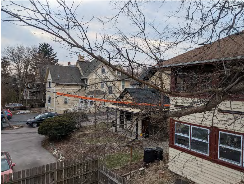
View of rear of 1213-1221 Rutledge Street from rear of subject property
