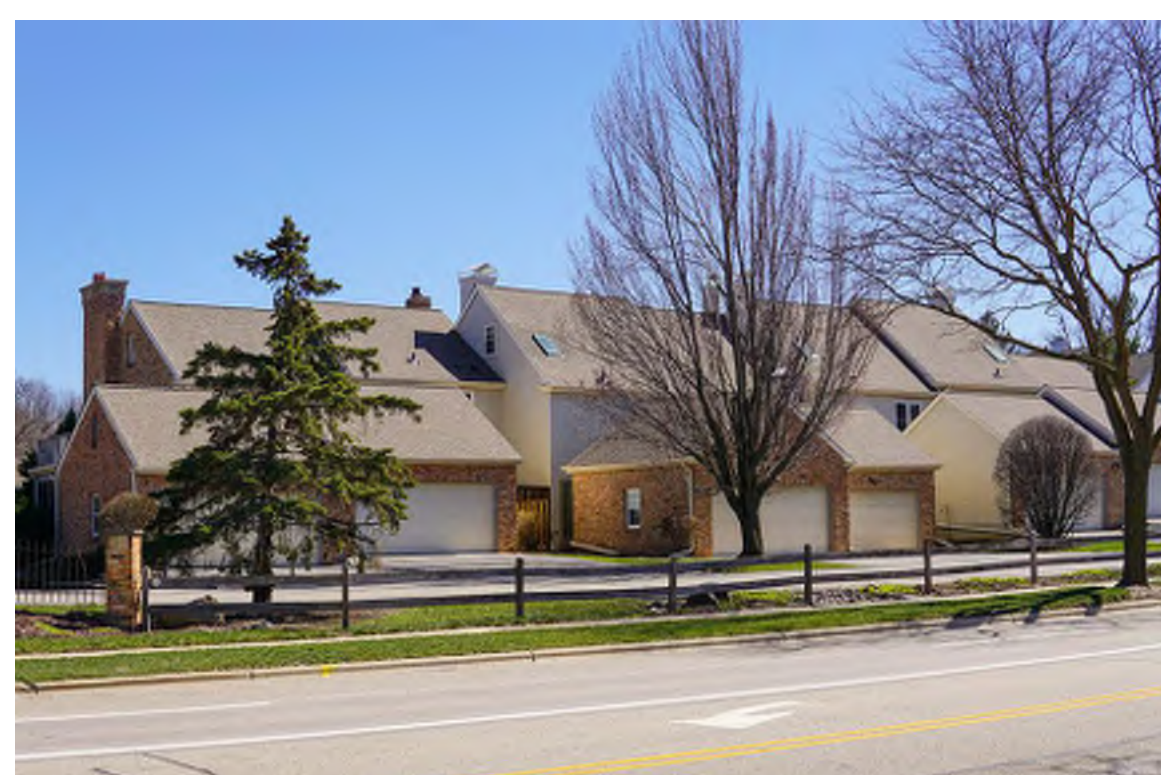
6925-6937 OLD SAUK ROAD WYNDEMERE CONDOMINIUMS
