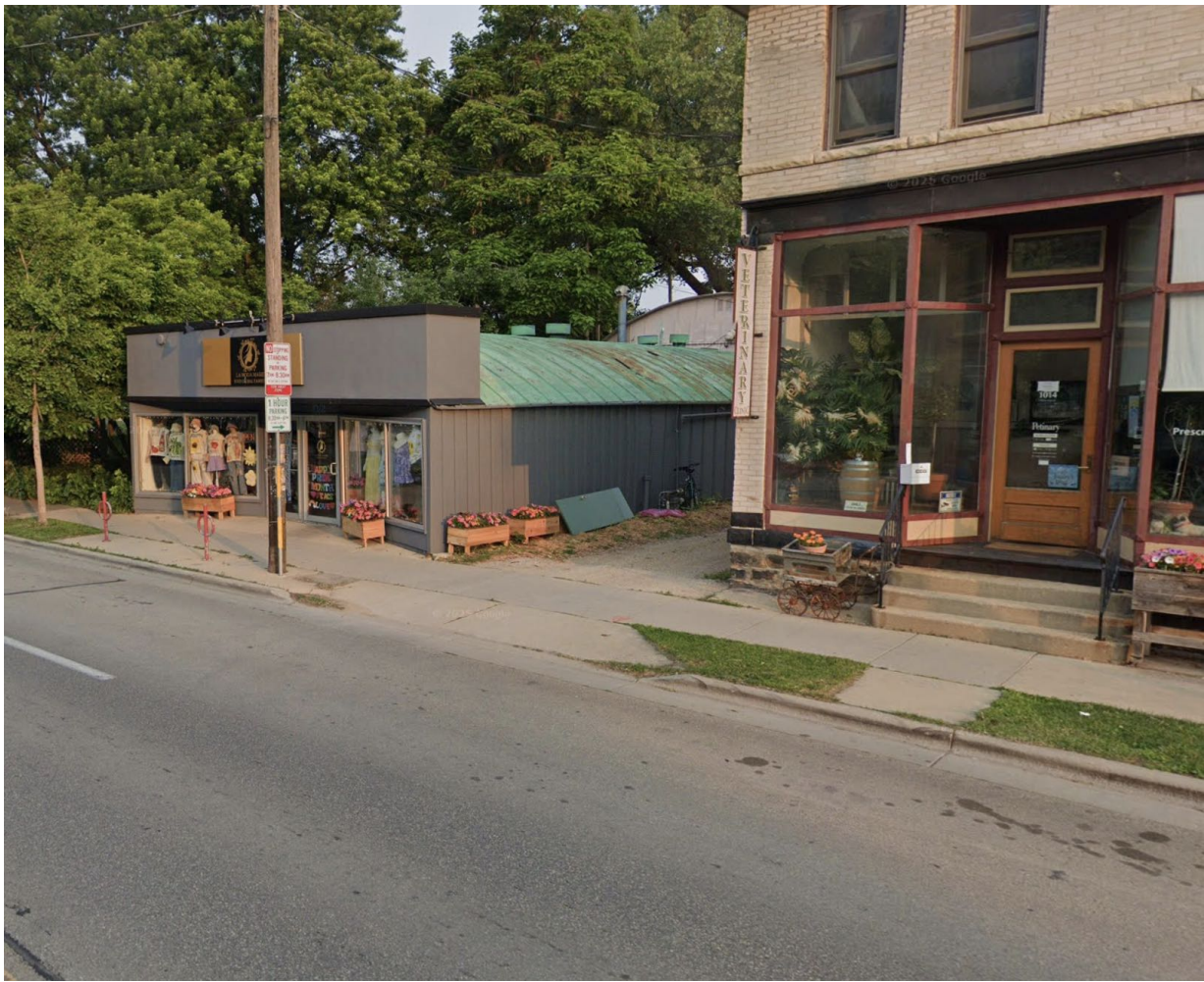
Fig. 3: Metal roof on Willy
