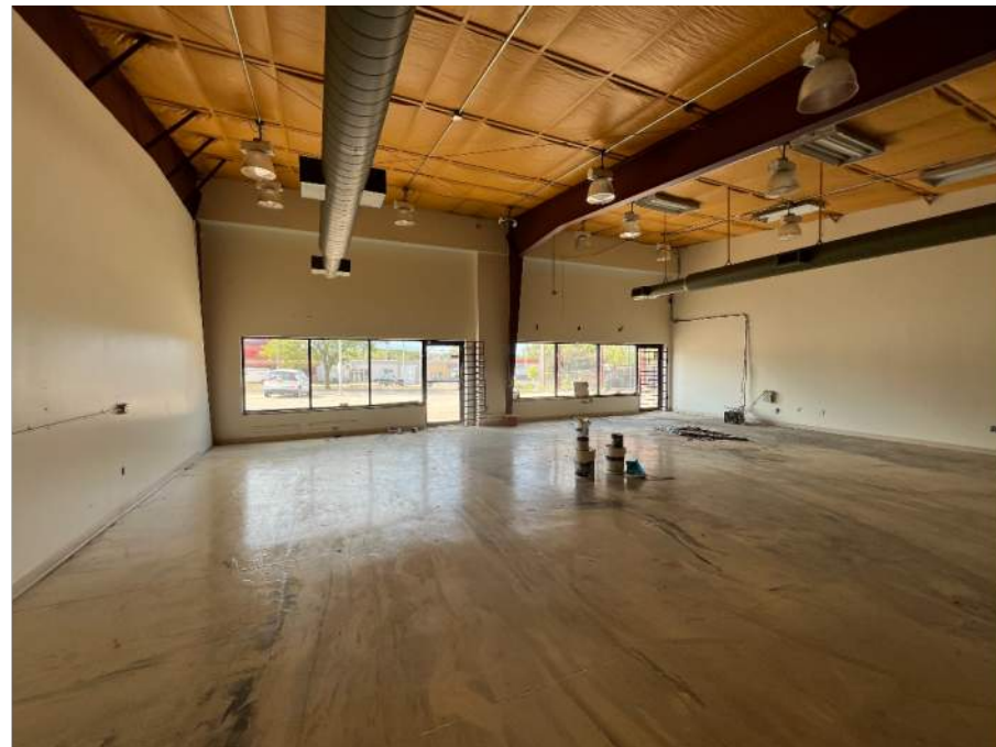
INTERIOR GROUND LEVEL
