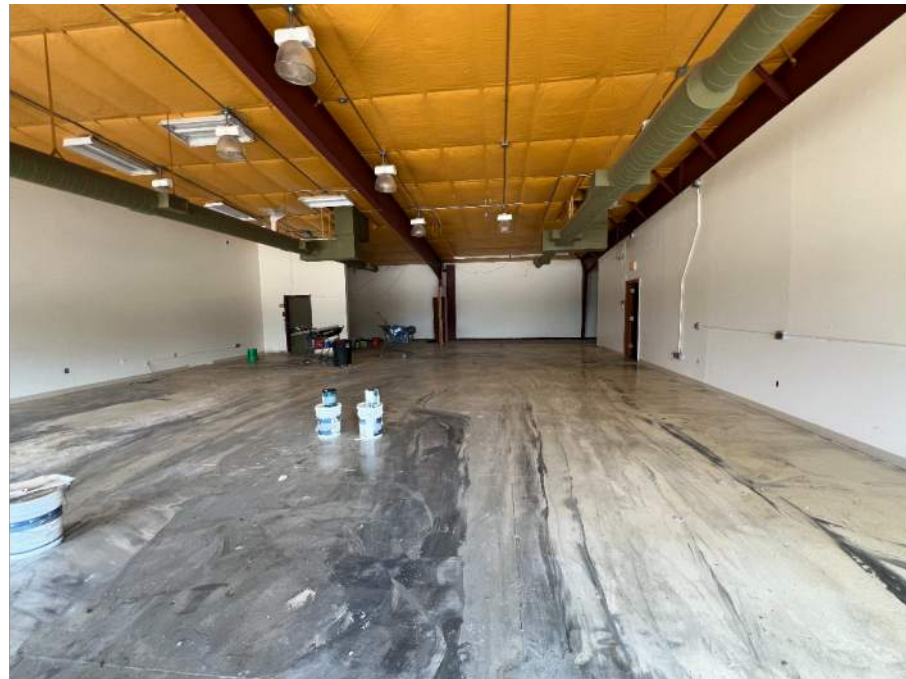
INTERIOR GROUND LEVEL
