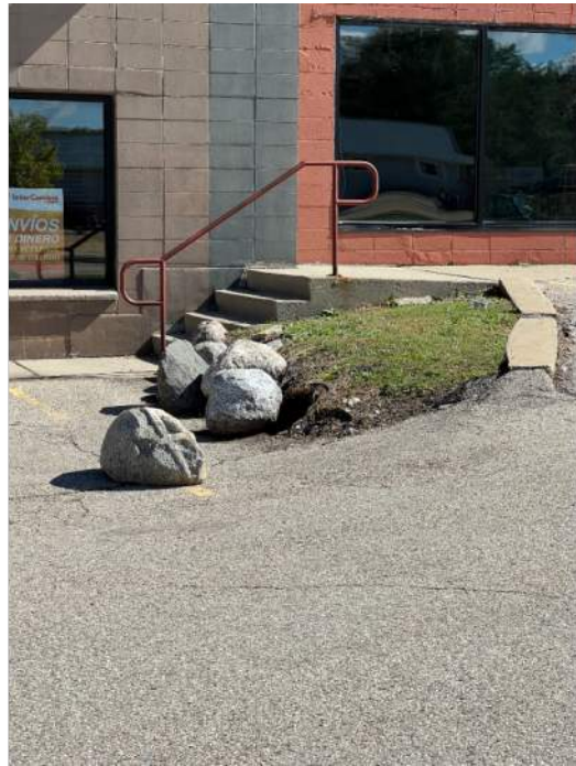
STAIRS AT BLDG FRONT
