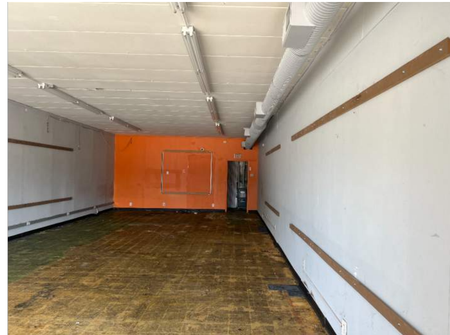
INTERIOR GROUND LEVEL
