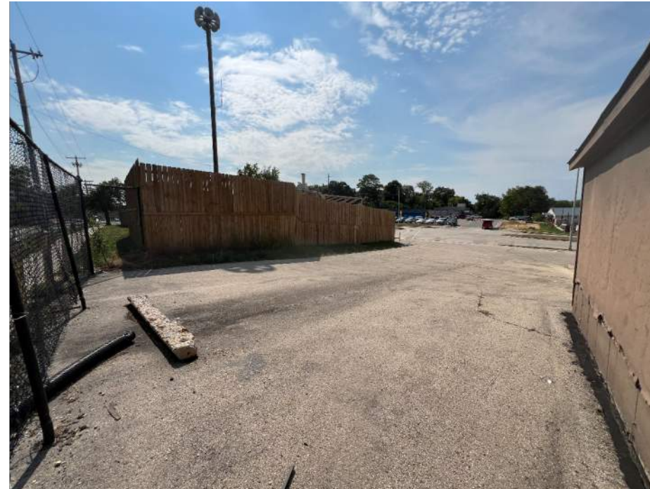
SOUTH END OF LOT LOOKING TOWARDS PARK ST & ADJACENT PROPERTY SCREENING FENCE
