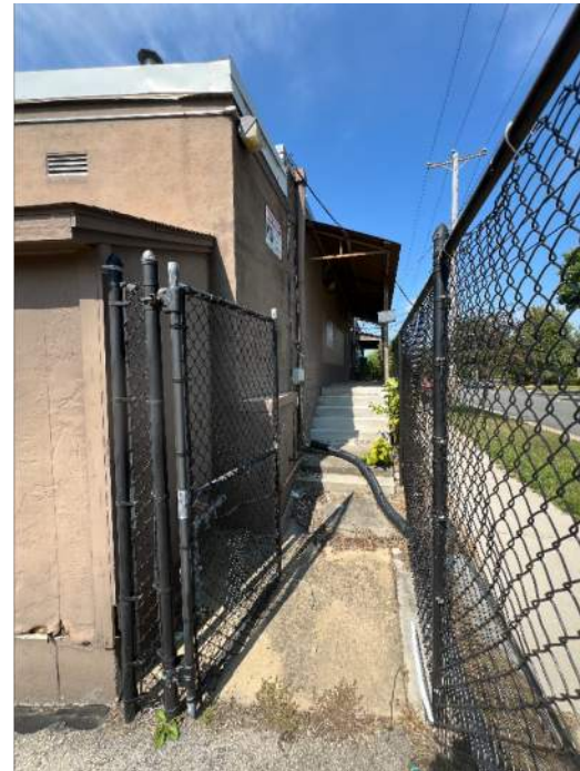
STAIRS AT BLDG SOUTH REAR
