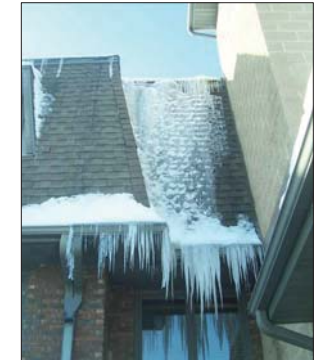
6 EXISTING BUILDING- 330 EAST IMAGE SCALE: NOT TO SCALE
