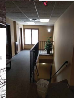
3 EXISTING BUILDING- 330 INTERIOR IMAGE SCALE: NOT TO SCALE
