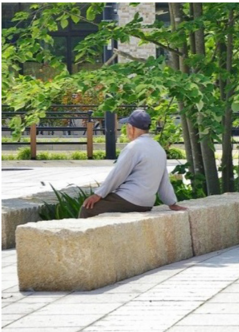
MATERIAL The stone plinths are thought to be limestone elements cut to shape with a smooth tops and rock-faced vertical faces.
