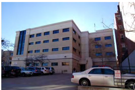
Parking Lot North Butler Street
