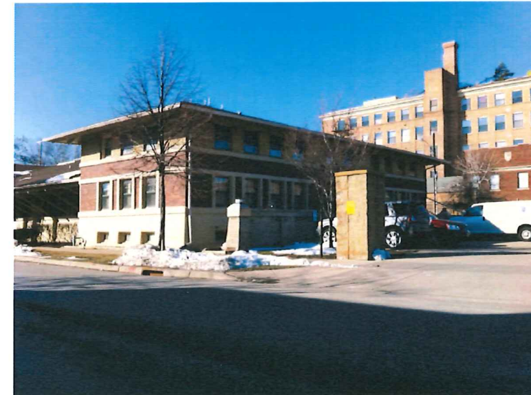
ADJACENT BUILDING ON E MIFFLIN STREET
