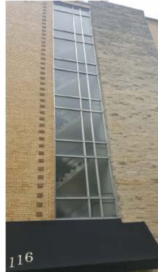
4 Existing Lobby Entry Canopy and Stair Tower Windows
