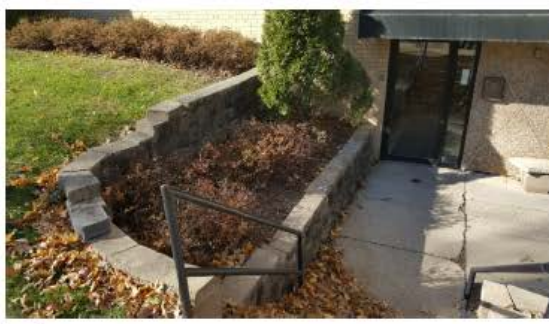
1 Existing Front Lobby Entry From Steps
