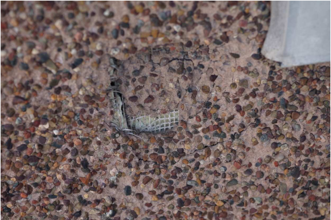
Fig. 21. Stucco damage
