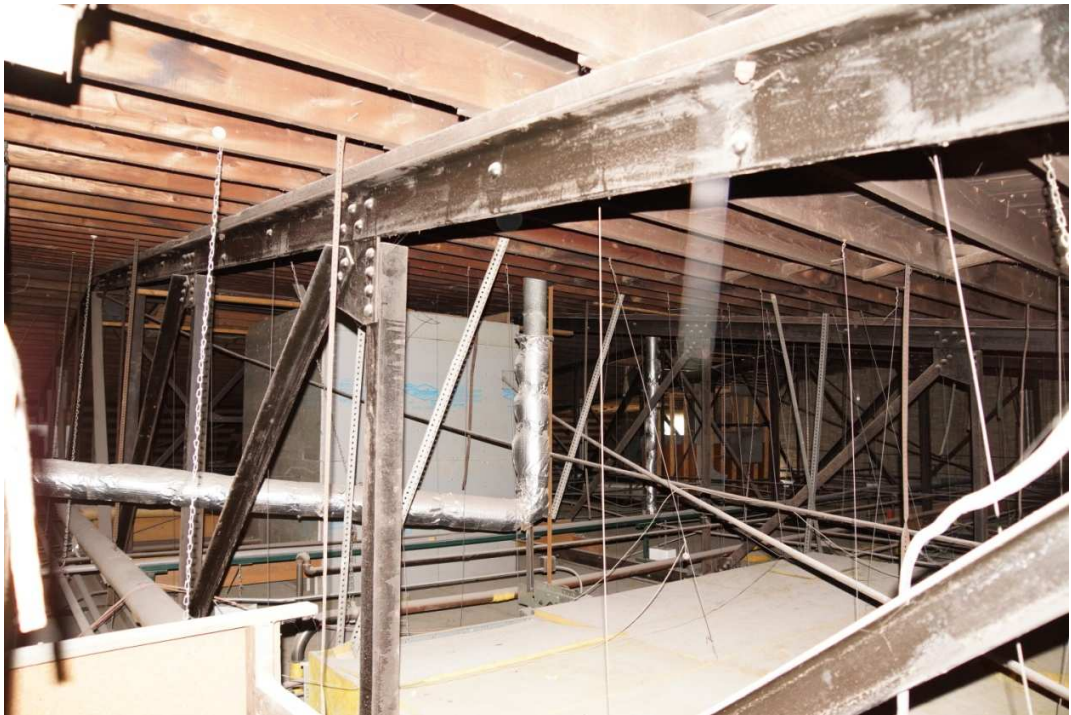
Fig. 3. Steel Roof Trusses
