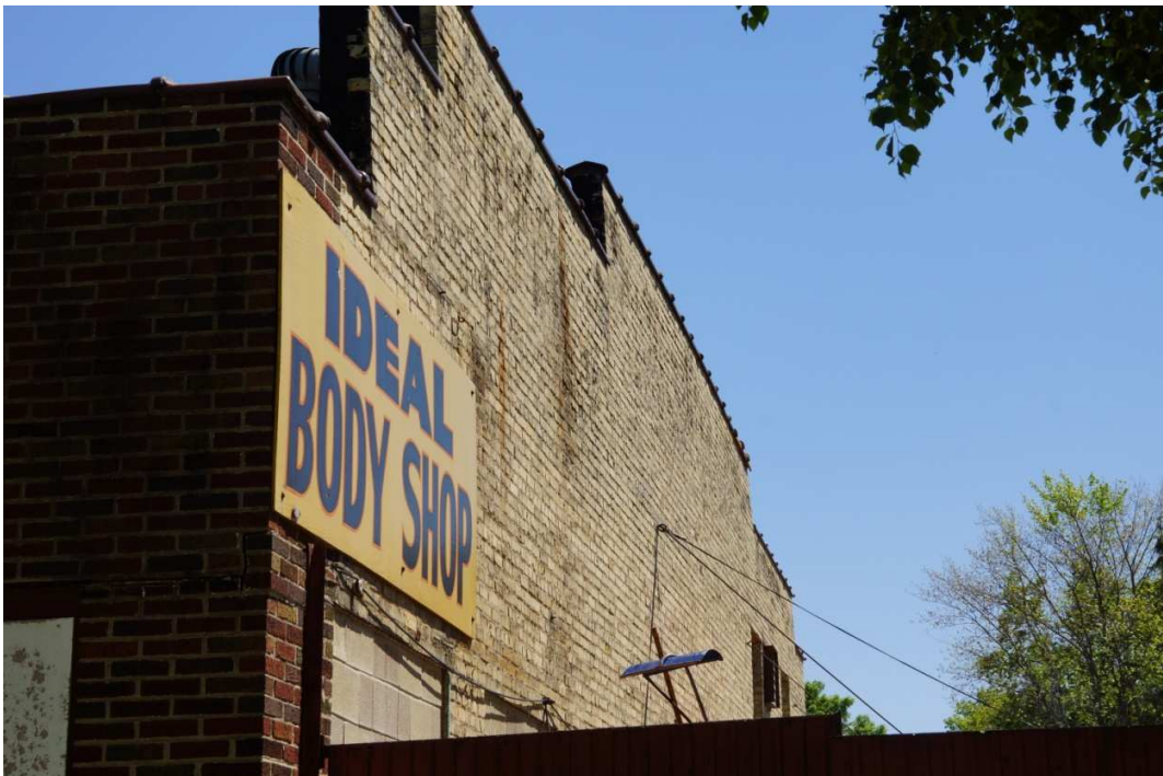
Fig. 8. Wall at the Back
