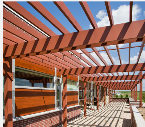
Madison Fire Station No. 12
