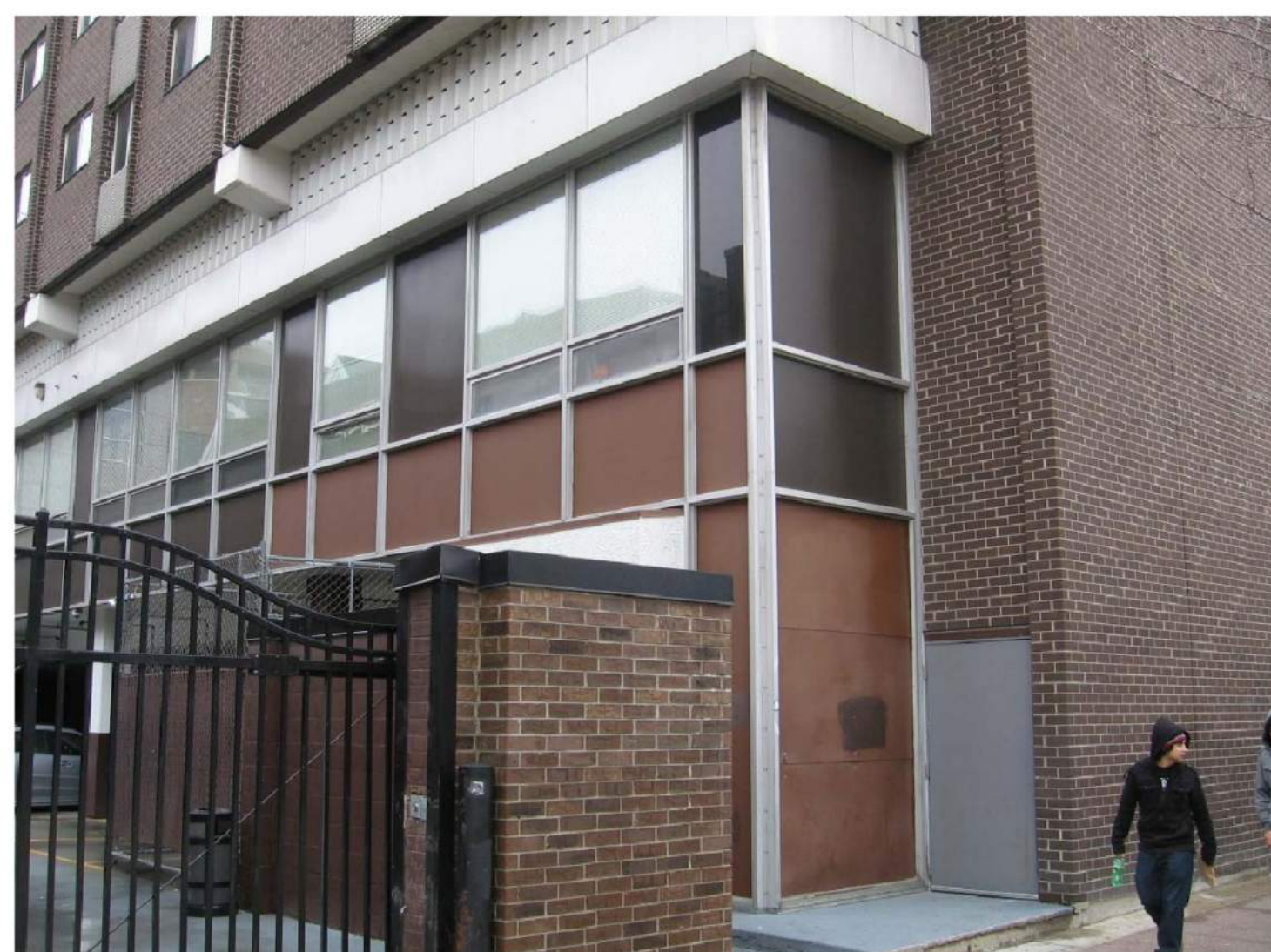
EXIT FROM EGRESS STAIR
