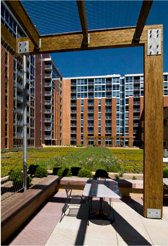
"Greenroof" with outdoor terrace
