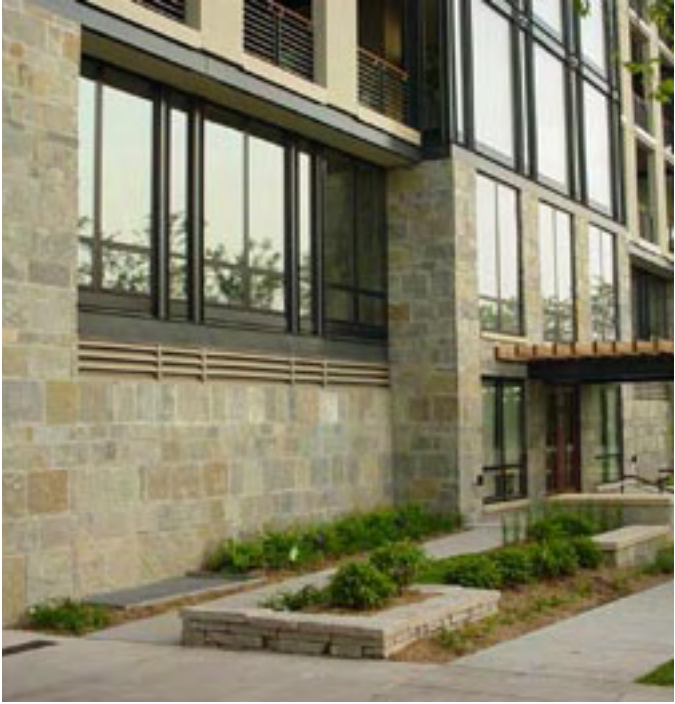
Dressed native limestone in ashlar or stacked patterns shall be incorporated into the design of publicly-visible façades
