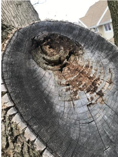
Picture of 14" pruning cut with decay on east side of scaffold A.
