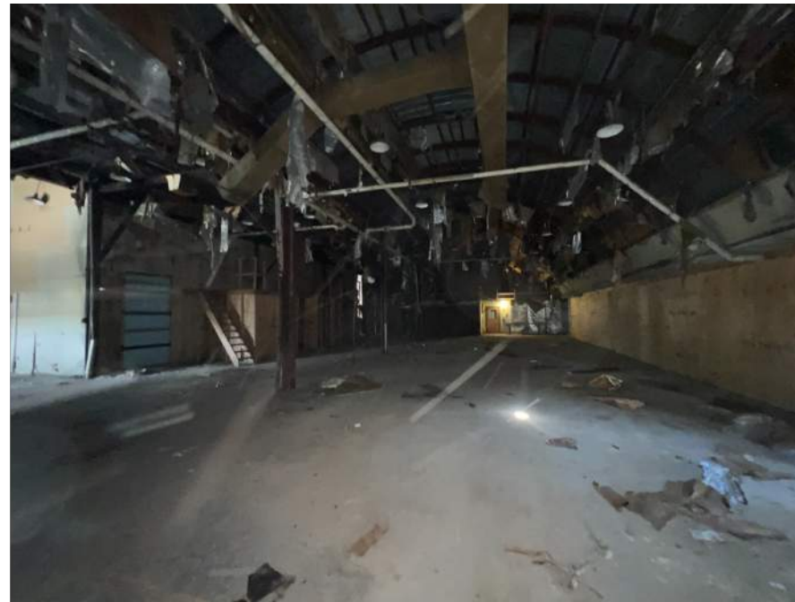
QUONSET STRUCTURE INTERIOR
