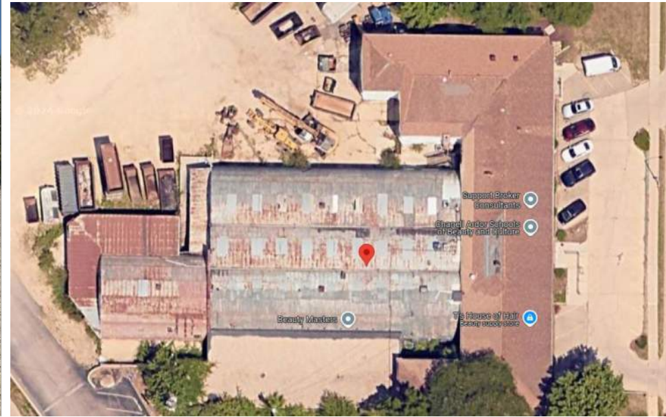
AERIAL VIEW OF STRUCTURE
