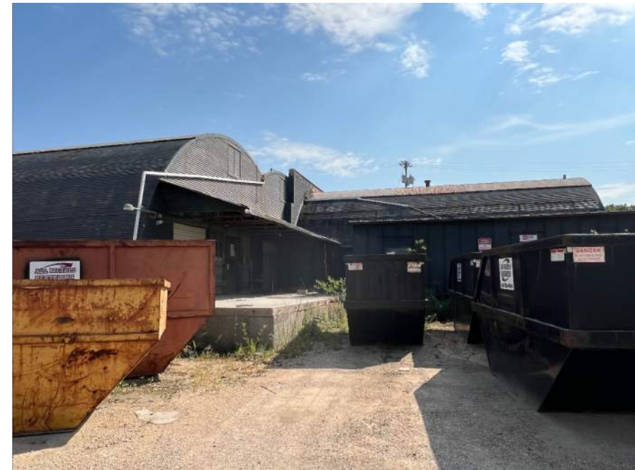
QUONSET STRUCTURES AT REAR OF BUILDING
