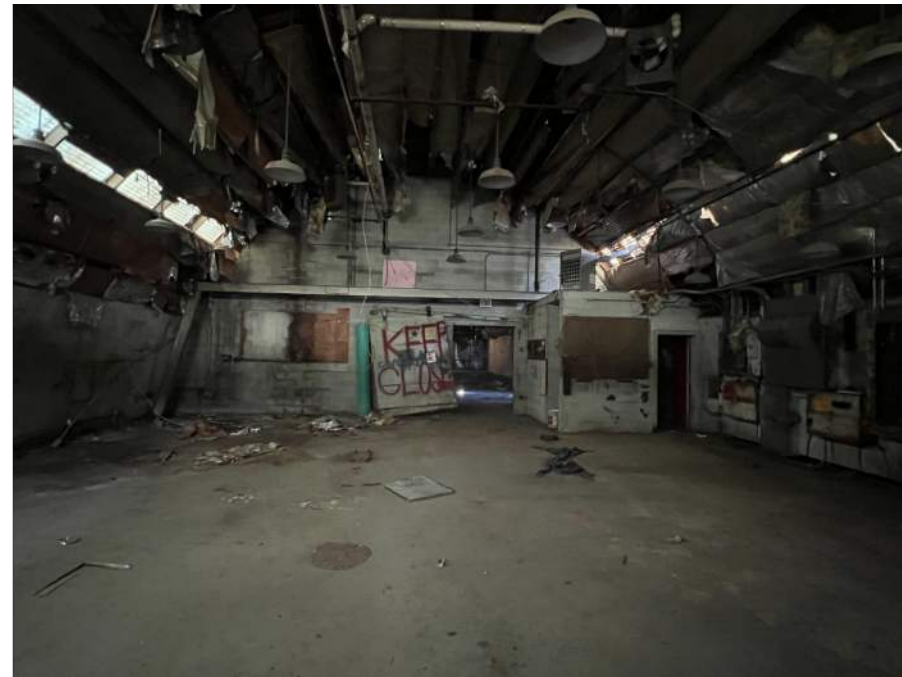
QUONSET STRUCTURE INTERIOR
