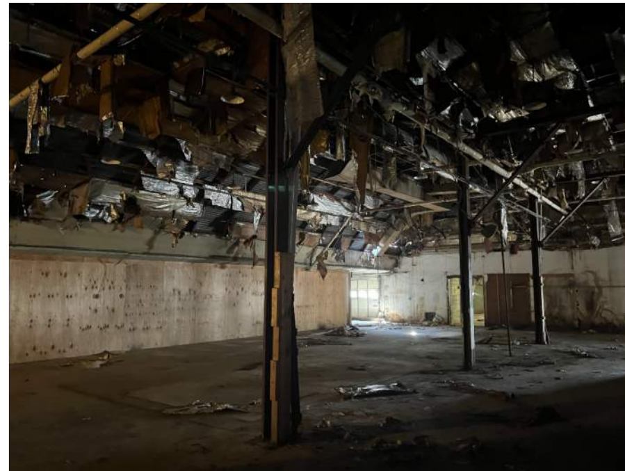
QUONSET STRUCTURE INTERIOR
