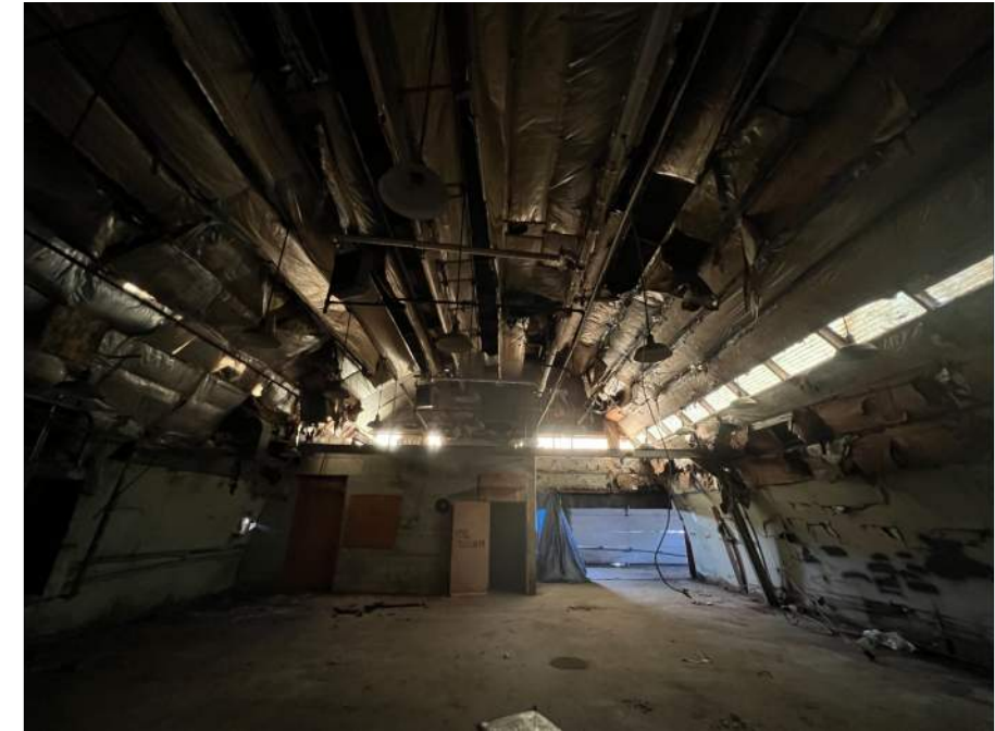
QUONSET STRUCTURE INTERIOR
