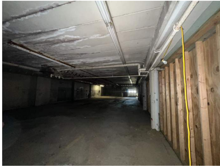
WAREHOUSE STRUCTURE INTERIOR
