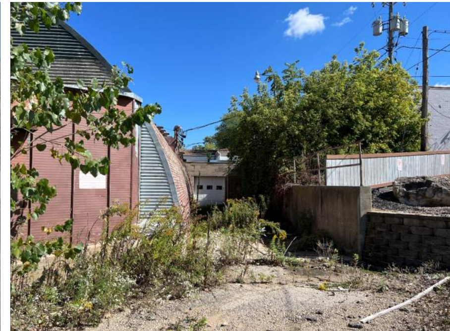
QUONSET AND WAREHOUSE STRUCTURES AT REAR OF BUILDING
