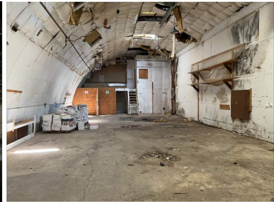
QUONSET STRUCTURE INTERIOR
