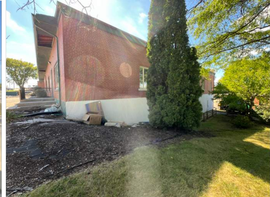
NORTH WALL VIEW FROM SOUTH PARK STREET
