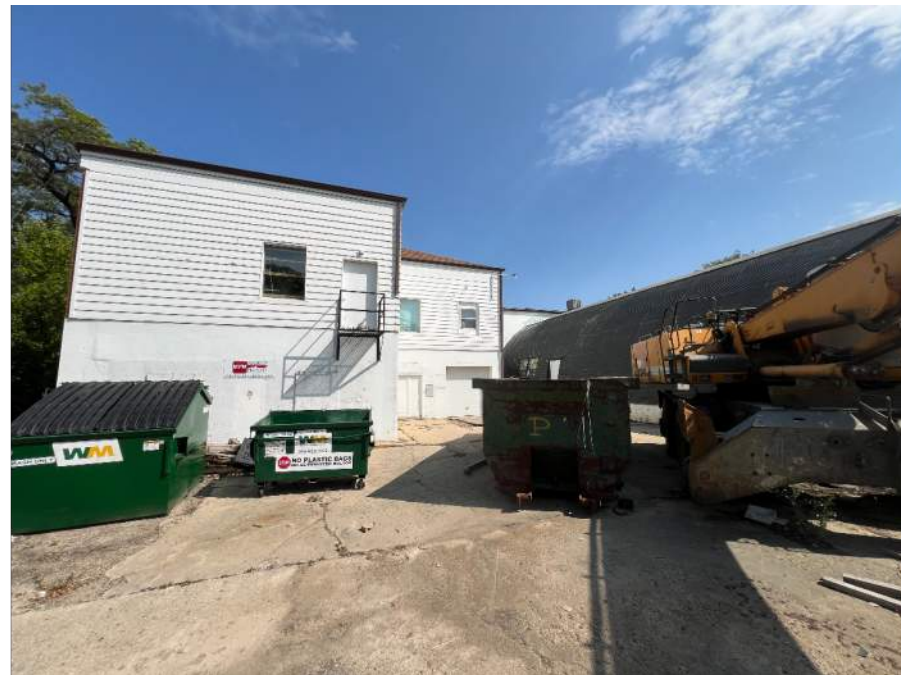
REAR VIEW AT NORTH SIDE OF PROPERTY
