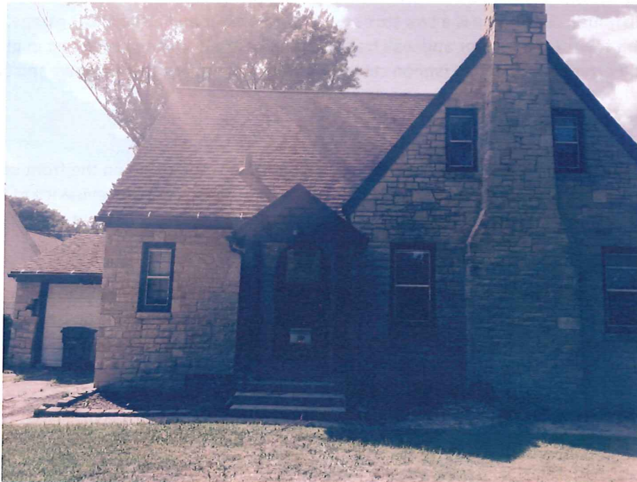
1. Exterior front view of home. (East elevation)
