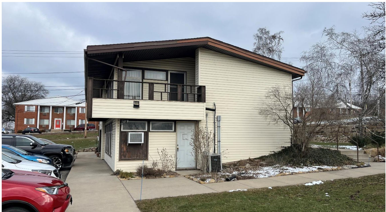
655 West Badger Road South side of two-story building to be demolished.
