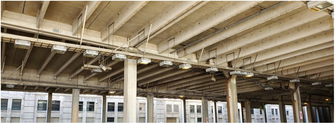
Existing Tunnel Lighting System to be Replaced
