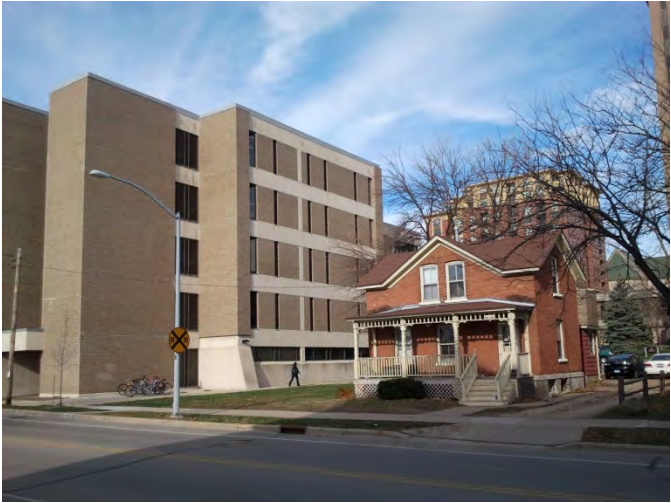
BUILDINGS WEST OF SITE (ALONG DAYTON STREET)
