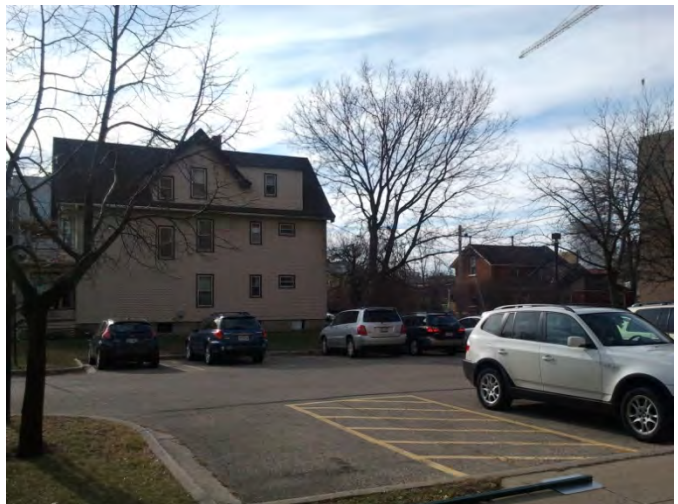
PROJECT SITE FROM THE NORTH - UW LOT #92
