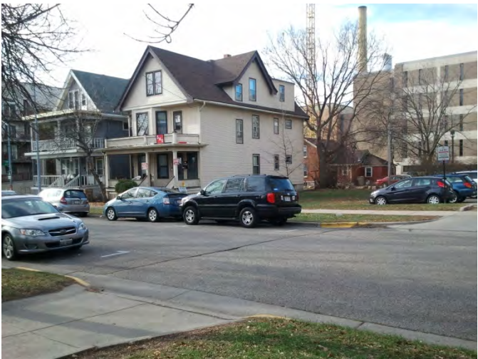
PROJECT SITE FROM NORTHEAST
