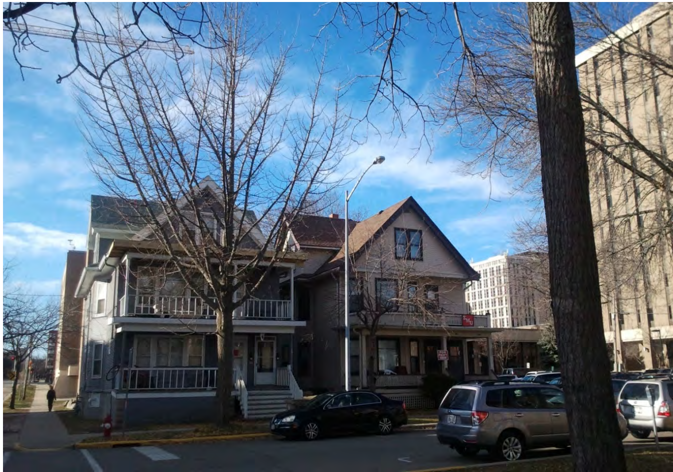
EXISTING STRUCTURES ON THE PROJECT SITE - (2) THREE STORY RENTAL BUILDINGS
