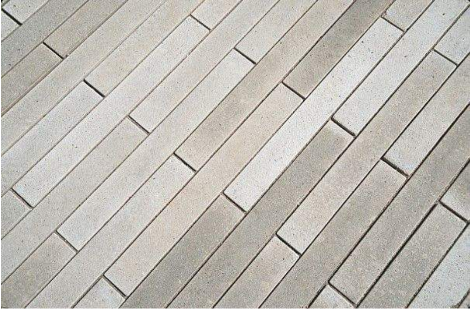
WALKING SURFACE SMALL SCALE RUNNING BOND PATTERN
