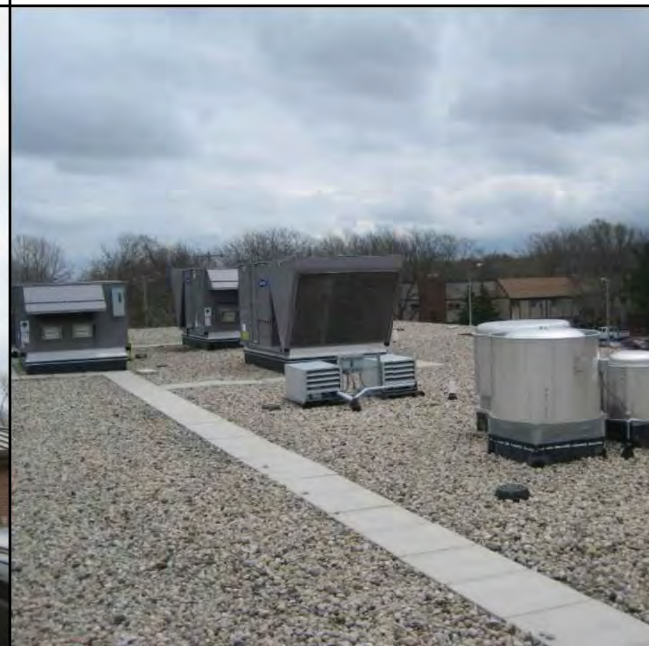
EXISTING BUILDING ROOFTOP
