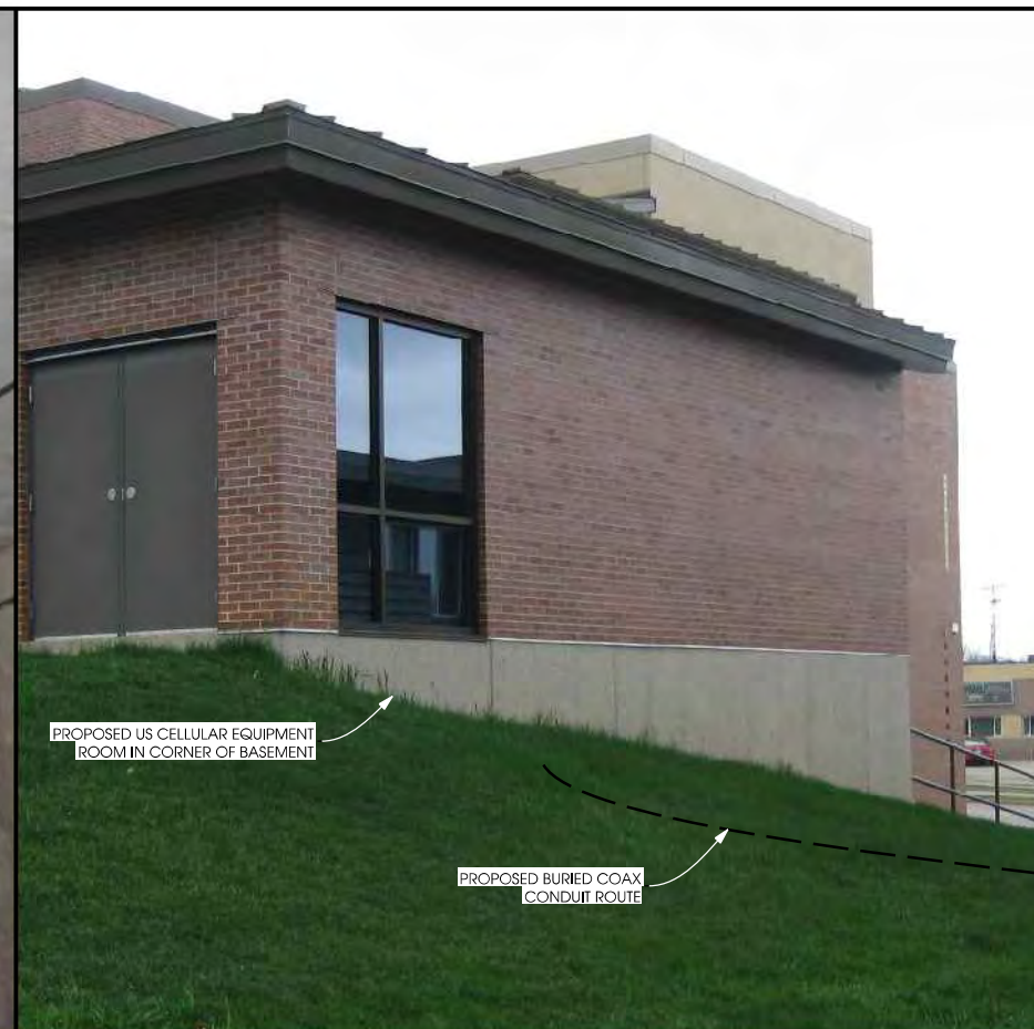
OUTSIDE EQUIPMENT ROOM
