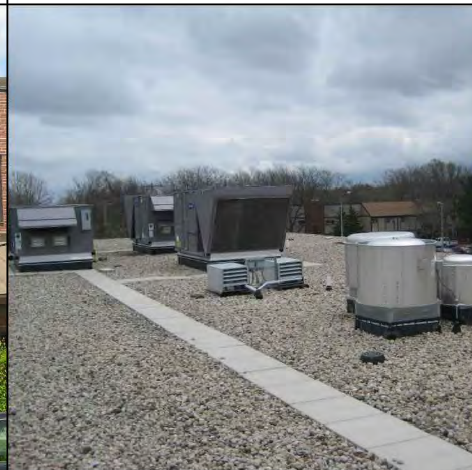
EXISTING BUILDING ROOFTOP
