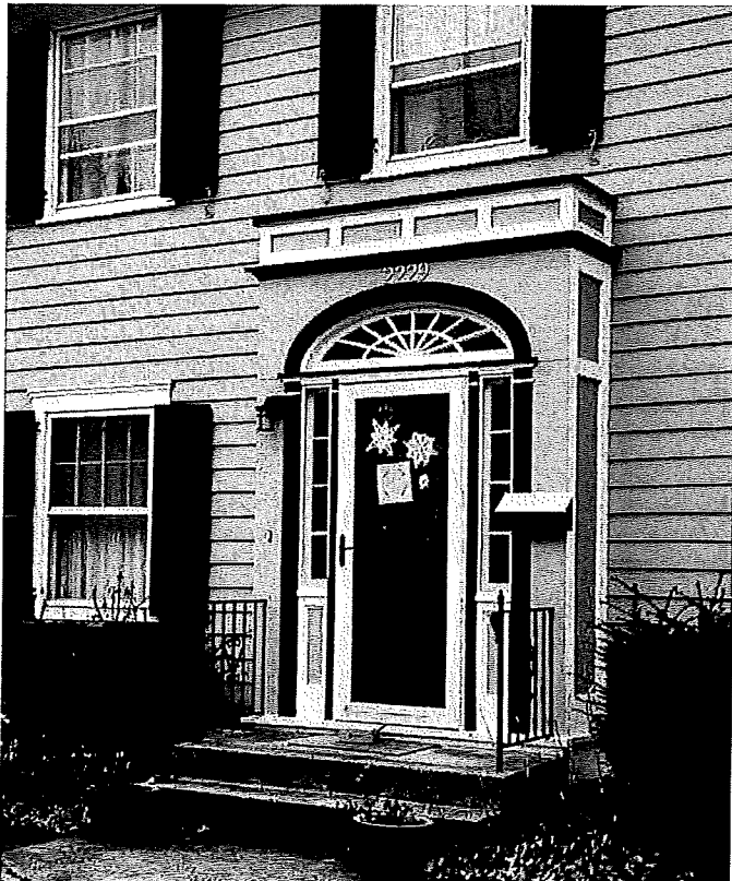
Front entrance looking southeast. 2229 Eaton Ridge, 2023.
