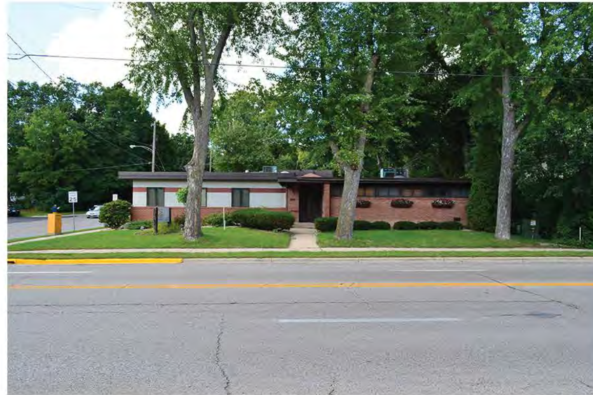
Existing Building along Monroe Street
