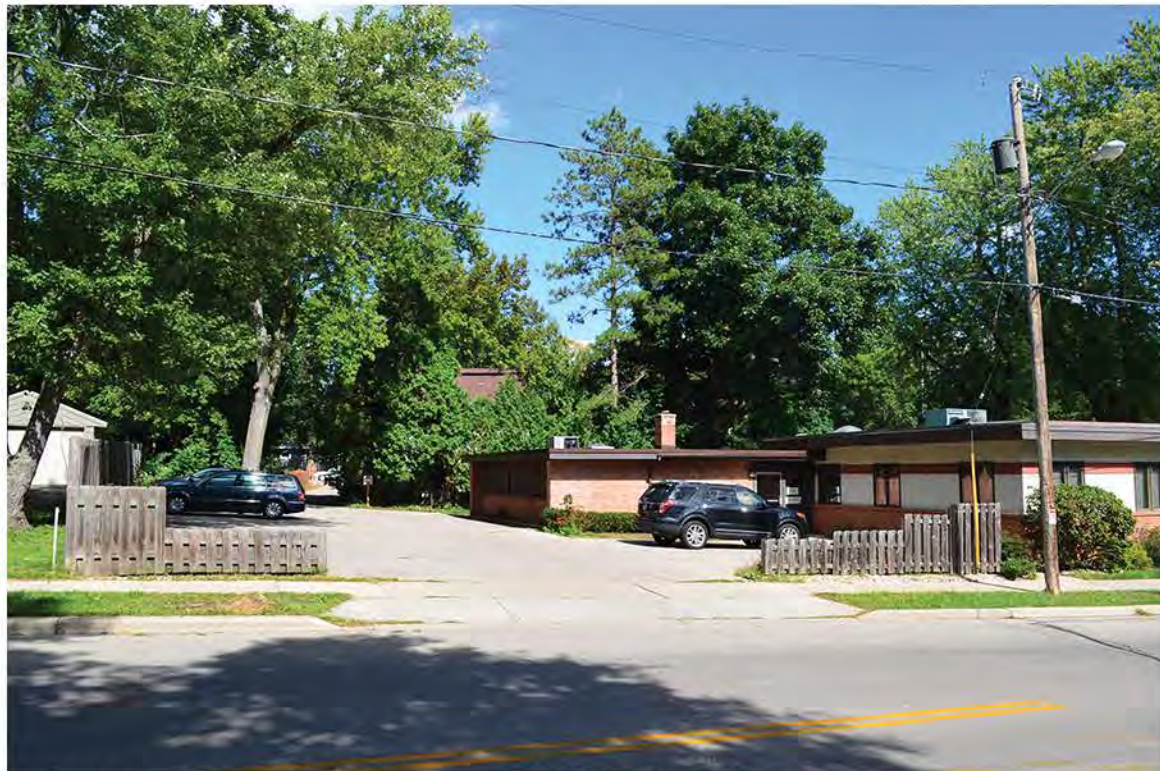
Existing Building parking accessed off of Glenway Street
