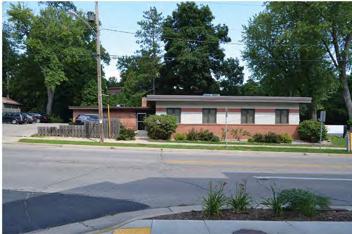
Existing Building along Glenway Street
