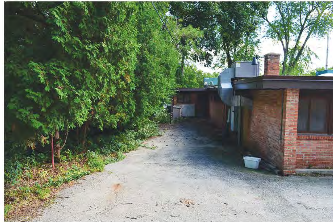
Existing Building adjacent to Arbor House property
