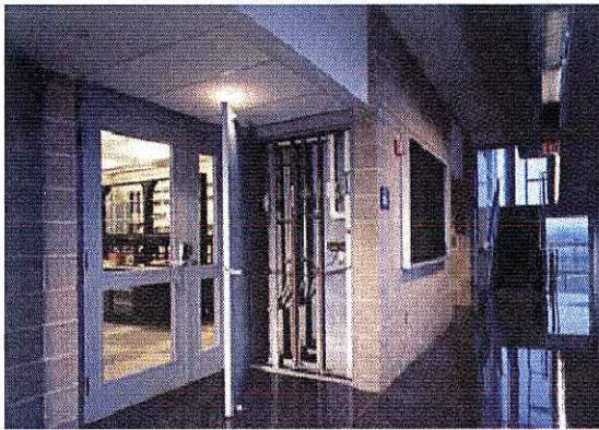
EASE OF ACCESS TO UTILITIES
