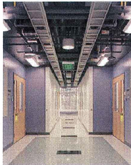
CORRIDOR ACCESS OVERHEAD
