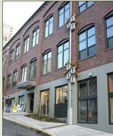
Rain drainage system, Seattle, WA
