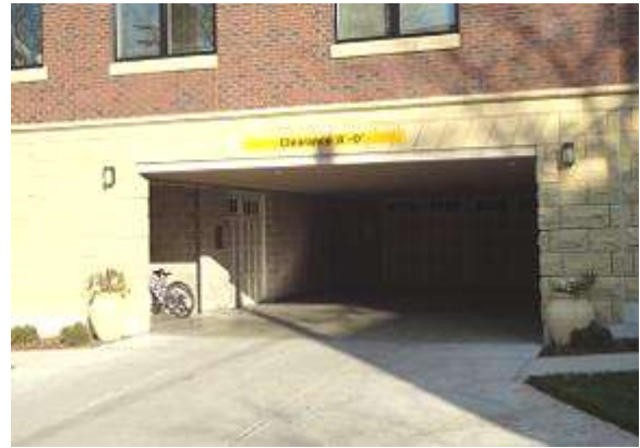
Recessed garage entrance on side street. Princeton Avenue, Madison.
