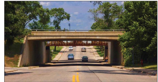
Current view of bridge underpasses
