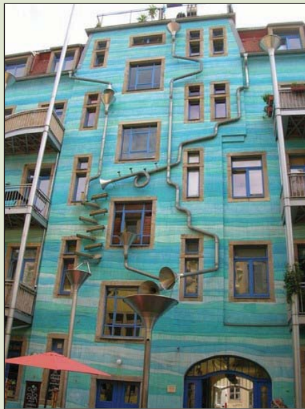
Rain drainage system Dresden, Germany
