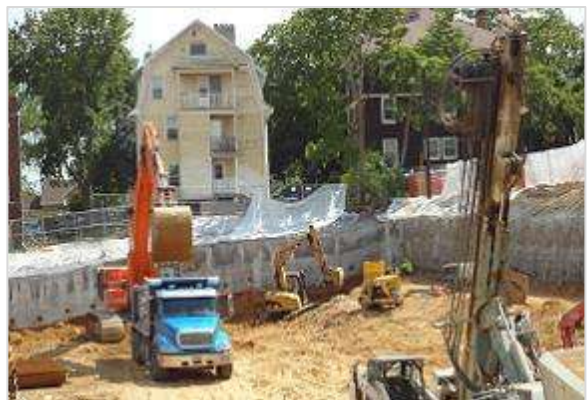
Construction of Brownlofts Apartments, University Avenue, 2013.
