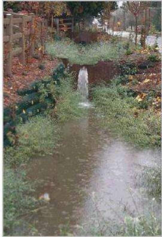
Storm water retrofit, Seattle, Washington.
