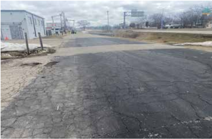
Commercial Av., near I-39 ALT (fair to good condition, crack, potholes, uneven surfaces)
