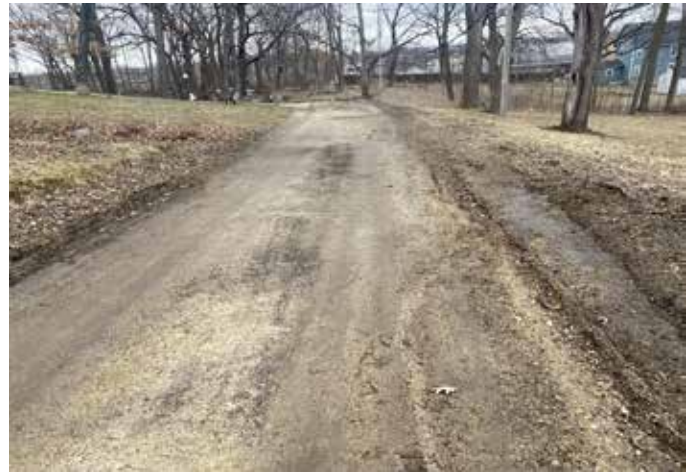
Ridgeway Ave, North of Grover Ave, (poor condition, untarred, water pooling surfaces)
