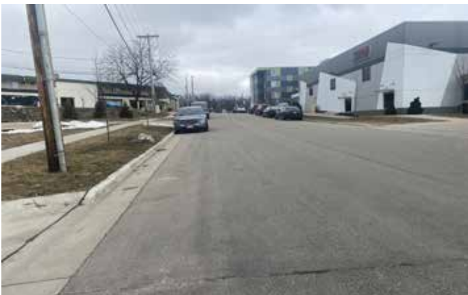
Rethke Ave (good condition)
