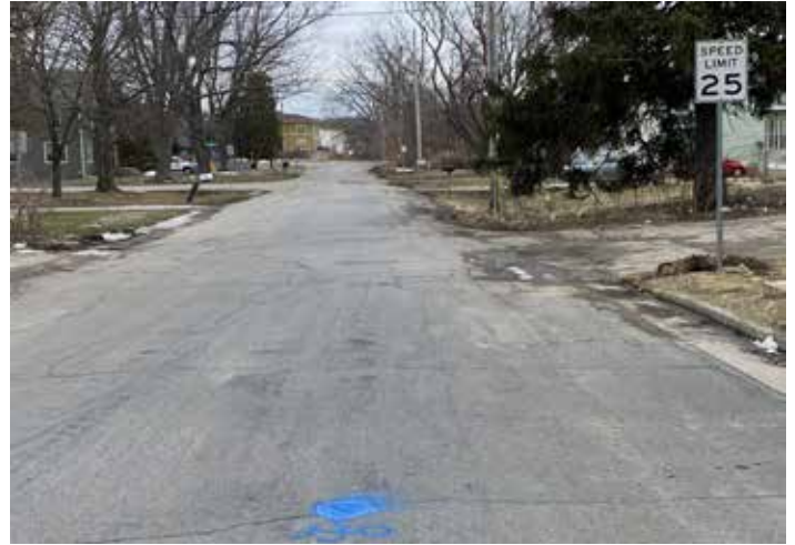
Schmedeman Ave off E Washington Ave (fair condition, crack, uneven surfaces)
