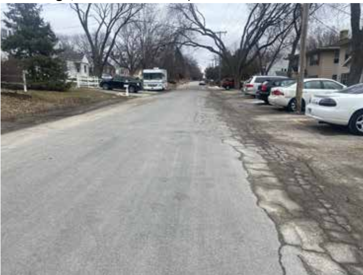
Ridgeway Ave, near E Washington Ave and Wright St, junction (fair condition, crack, no curb and drainage, uneven surfaces)
