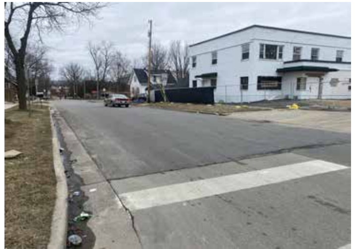
Schmedeman Ave off E Washington Ave (fair condition, crack, uneven surfaces)
