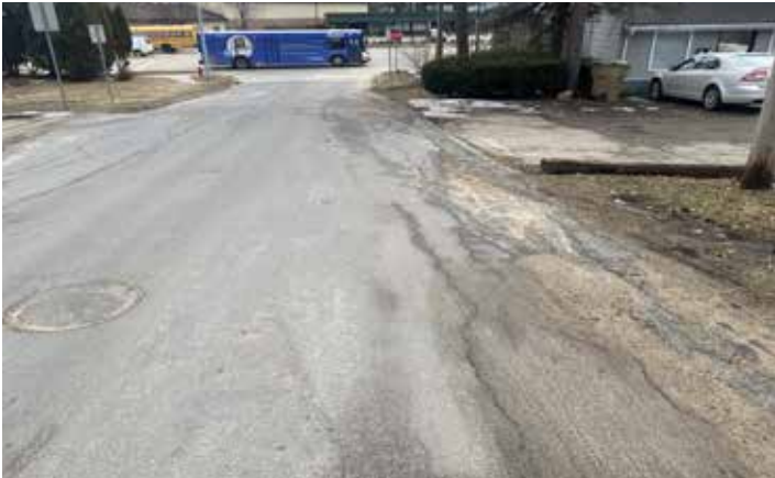
Carpenter Str, off E Washington Ave. (fair to poor condition, crack, uneven surfaces)
