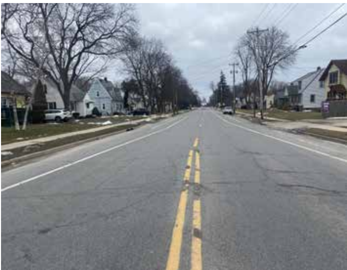
N Fair Oaks Ave, near E Washington junction (fair to good condition, minor crack)
