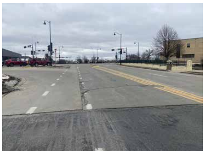
N Fair Oaks Ave, near E Washington junction (fair to good condition, minor crack)
