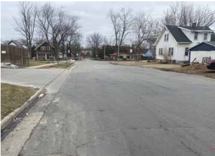
Schmedeman Ave off E Washington Ave (fair condition, crack, uneven surfaces)
