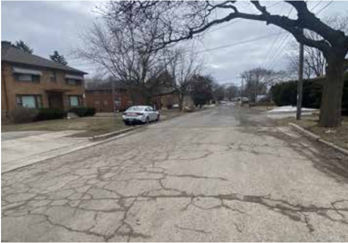
Pinecrest Dr, Near E Washington Ave, (fair condition, cracking, no gutter)
