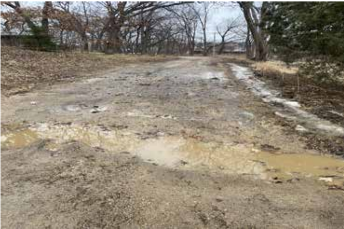
Ridgeway Ave, North of Grover Ave, (poor condition, untarred, water pooling surfaces)
