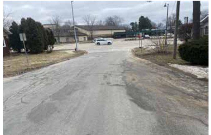
Carpenter Str, off E Washington Ave. (fair to poor condition, crack, uneven surfaces)
