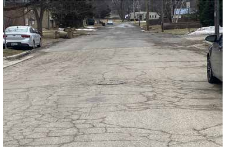
Pinecrest Dr, Near E Washington Ave, (fair condition, cracking, no gutter)
