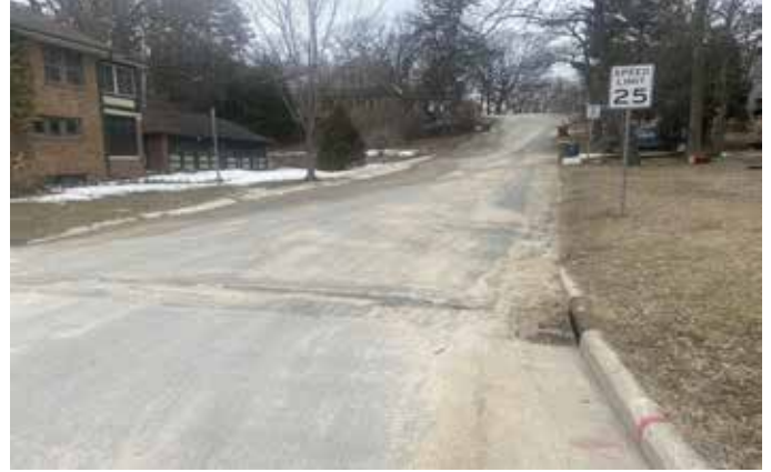
Grover St., near E Washington and Wright St. Junction (fair condition, some cracking and uneven surfaces)
