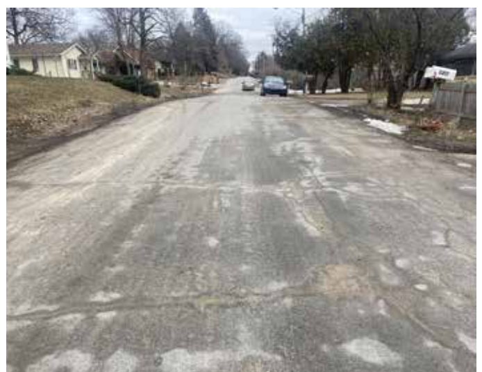
Ridgeway Ave, near E Washington Ave and Wright St, junction (fair condition, crack, no curb and drainage, uneven surfaces)
