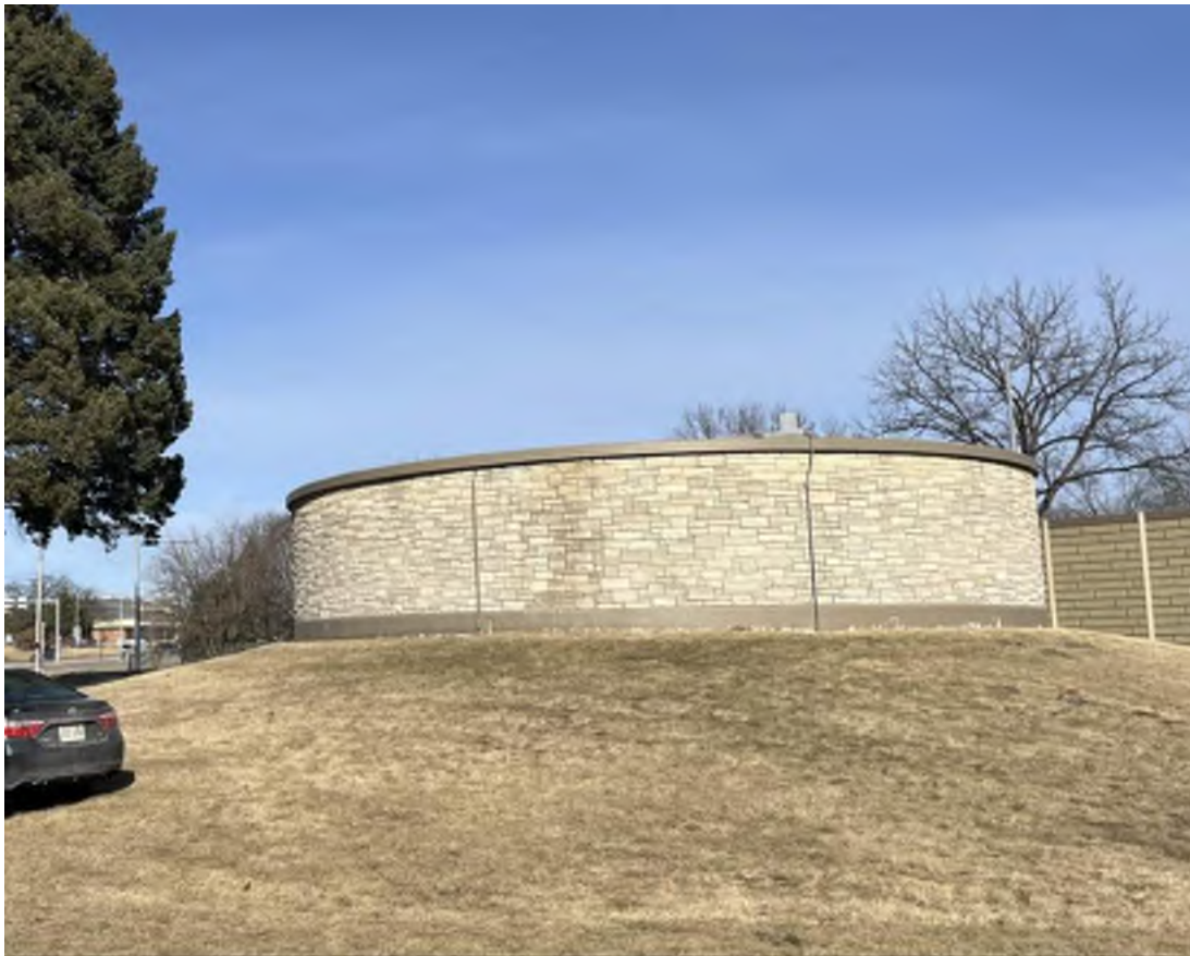
Existing Reservoir to be removed and replaced.
