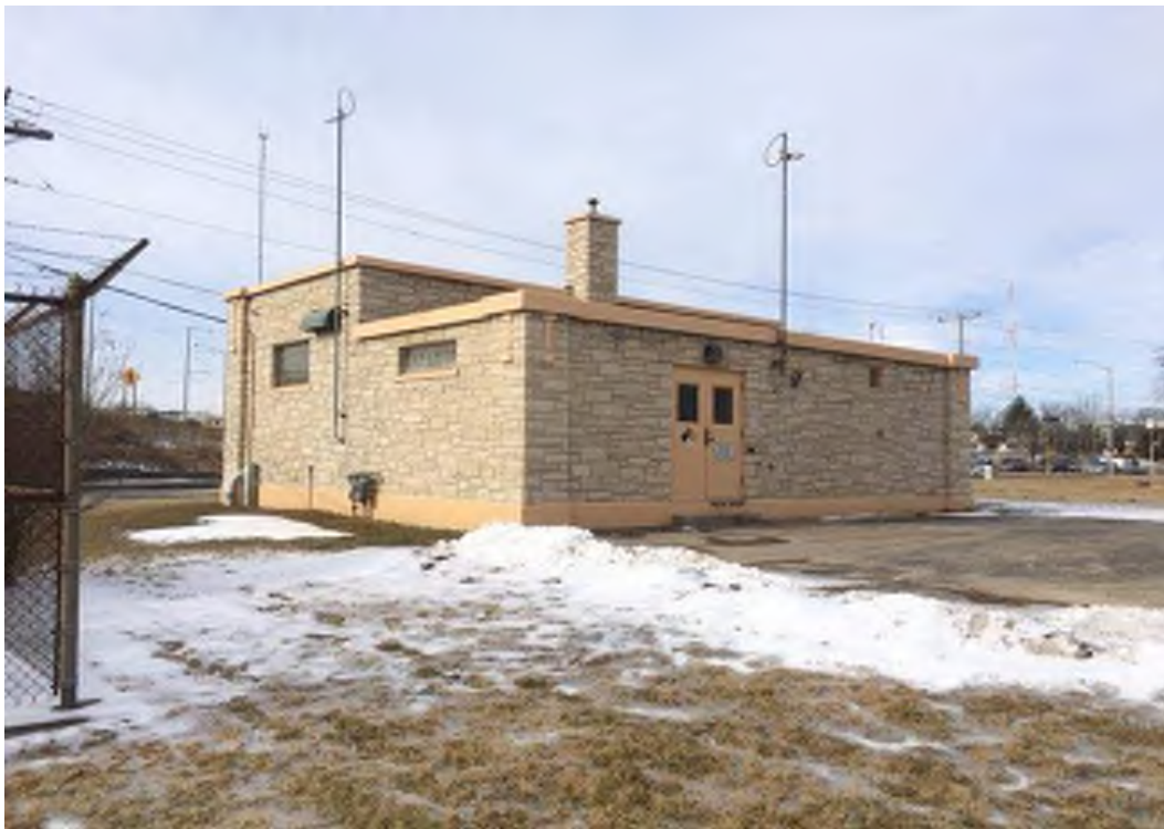
The rear of the existing Wellhouse.
