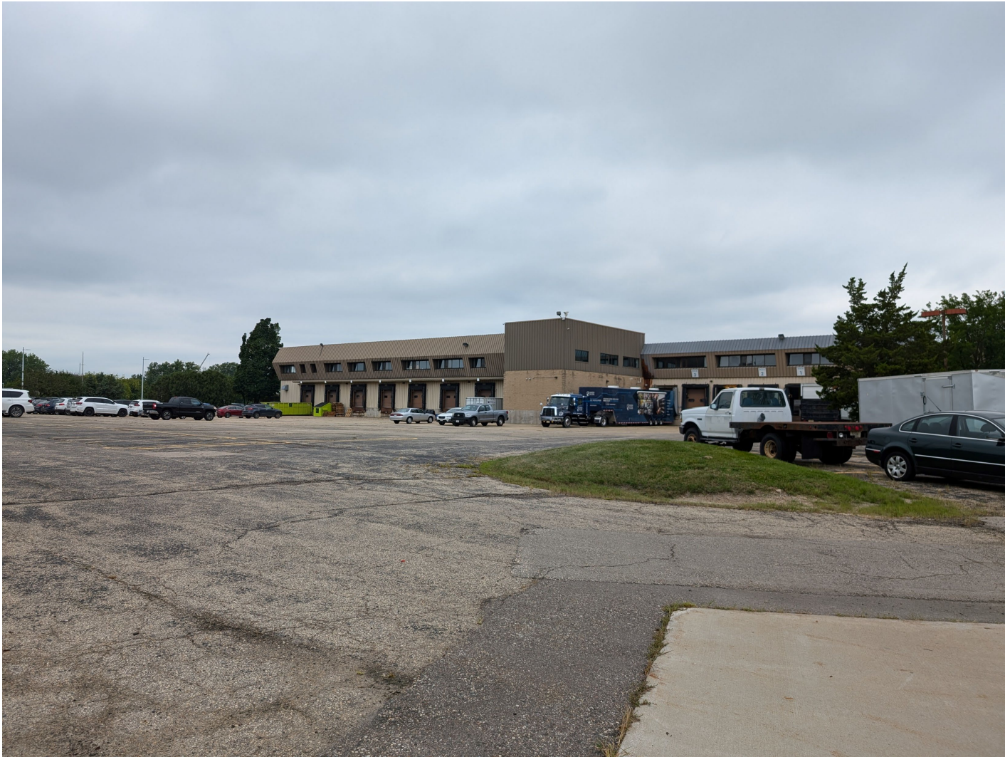
South Elevation, Compliant Location for Outdoor Storage
