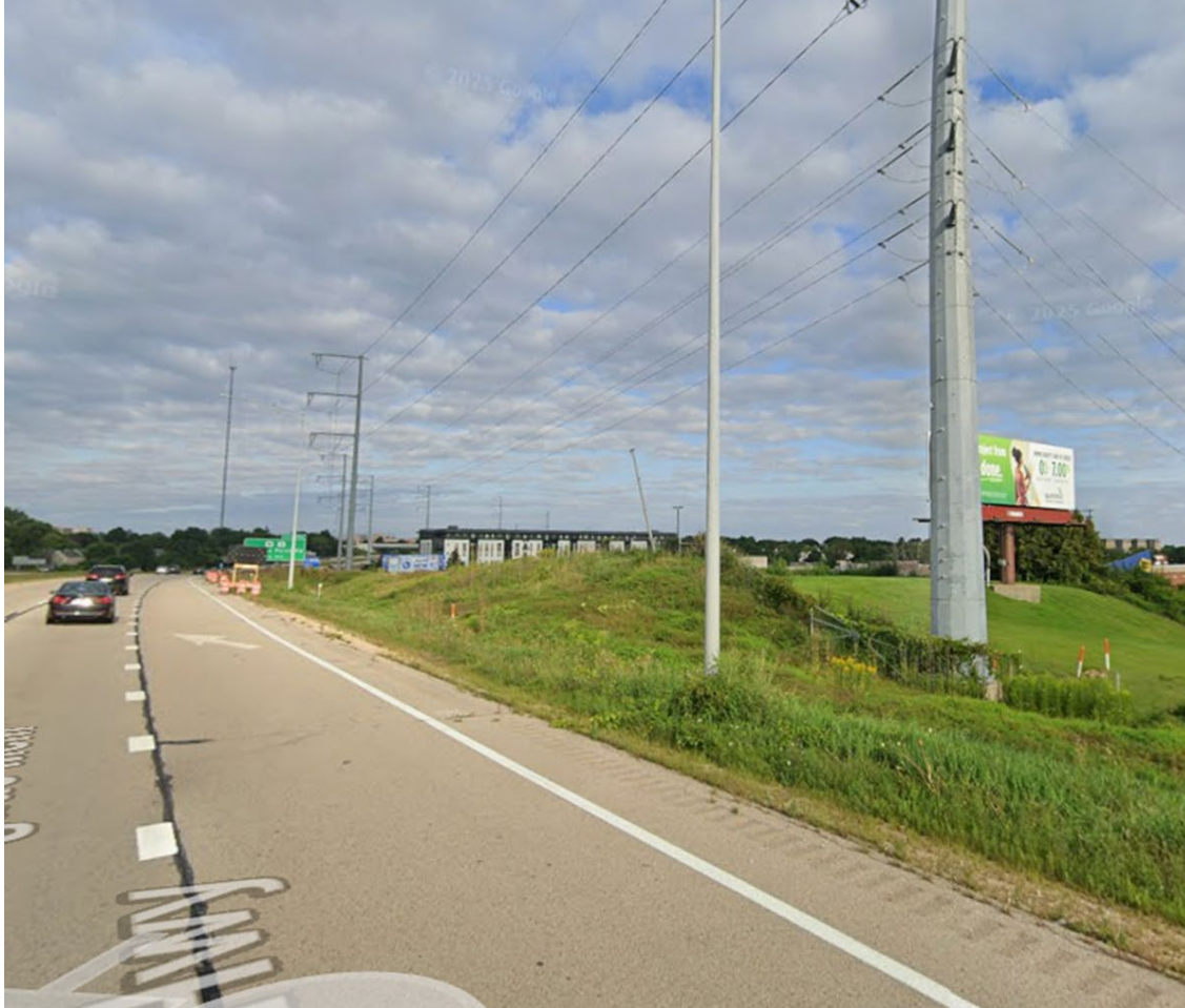
Looking west towards future route of path adjacent to W Beltline Hwy
