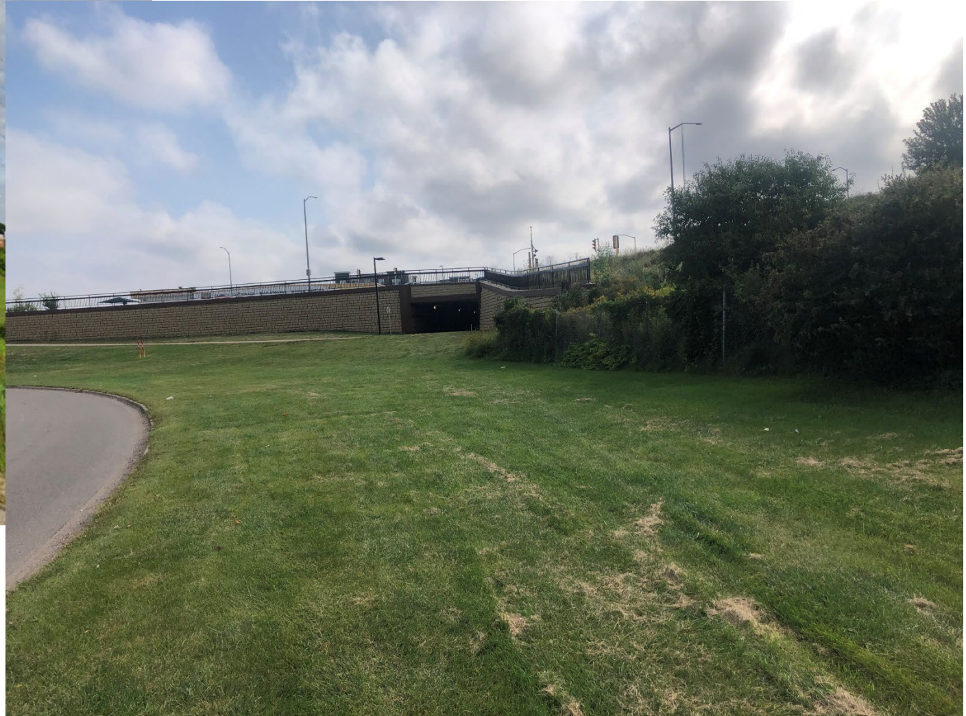
Looking west towards existing path underpass under S Gammon Rd, future path to connect to underpass
