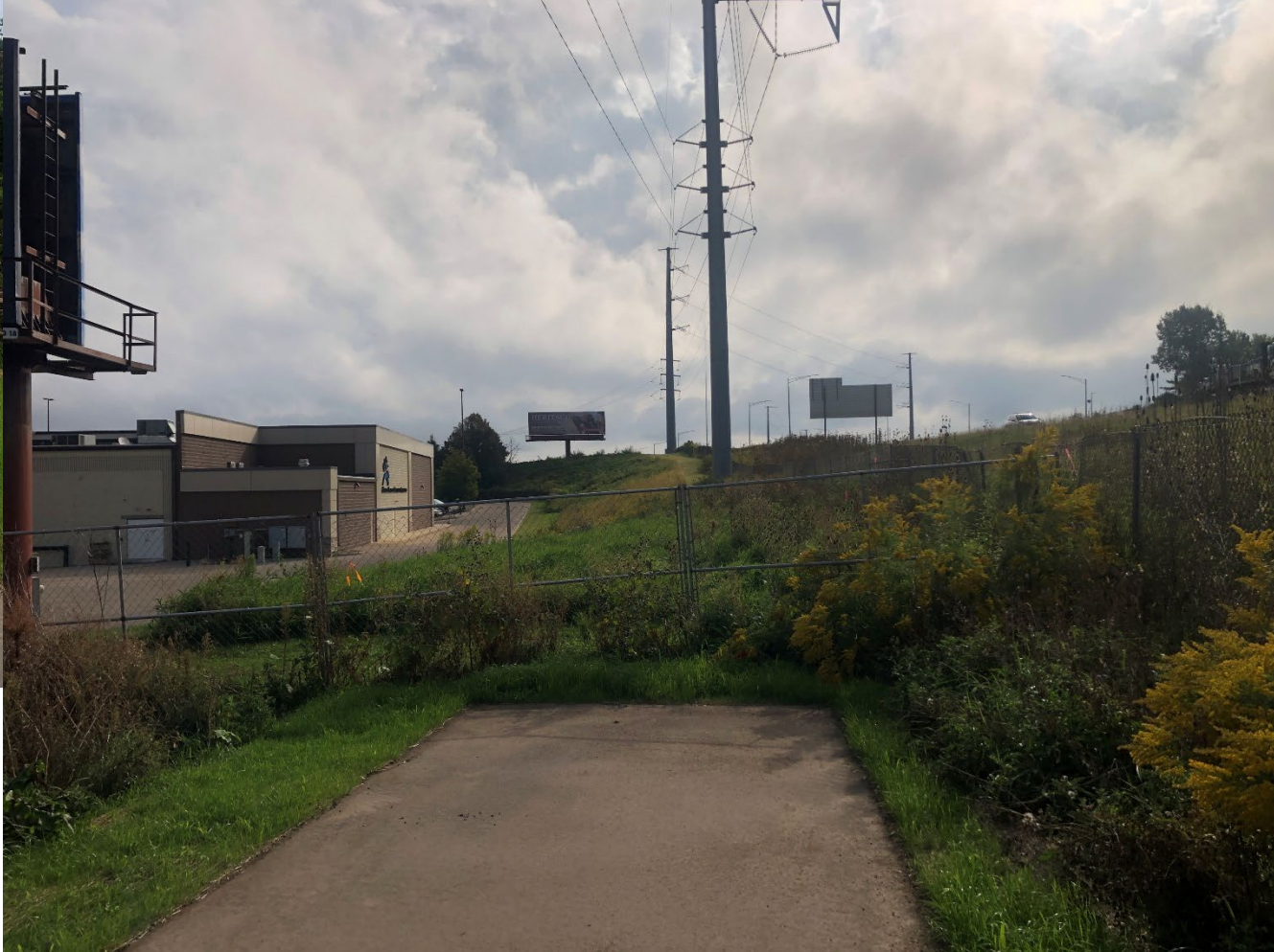
End of WTP: Phase 2a – Looking east towards future route for Phase 2b (this project), W Beltline Hwy on the right
