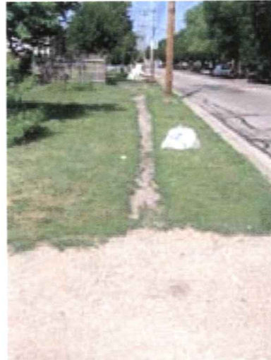
Badger Road Missing Sidewalk July 7, 2005
