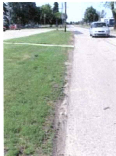
Perry Street Missing Sidewalk July 7, 2005
