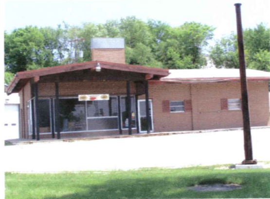
2421 South Park Street Vacant building, sagging eave trough May 25, 2003
