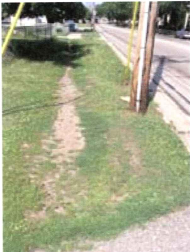
Missing Sidewalk Badger Road July 7, 2005
