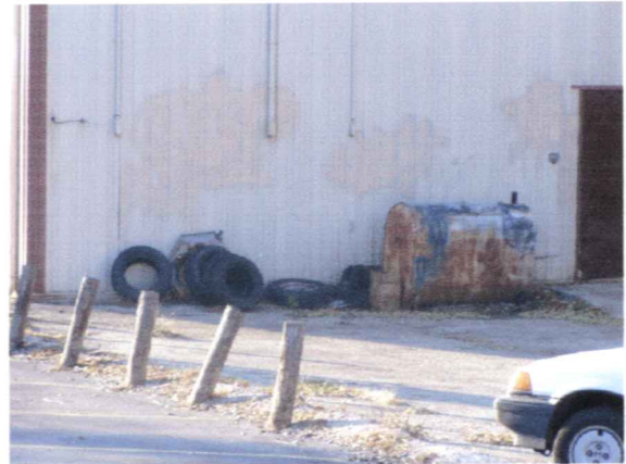
1817 South Park Street Trash, bent posts October 25, 2003
