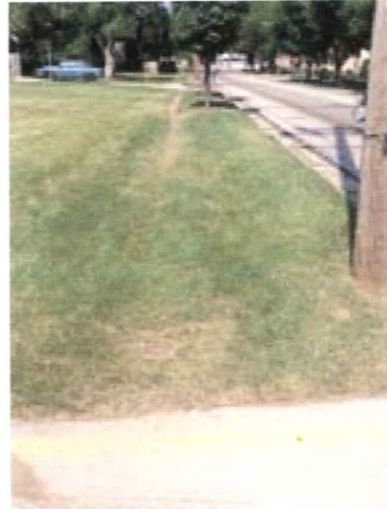
Badger Road Missing Sidewalk July 7, 2005
