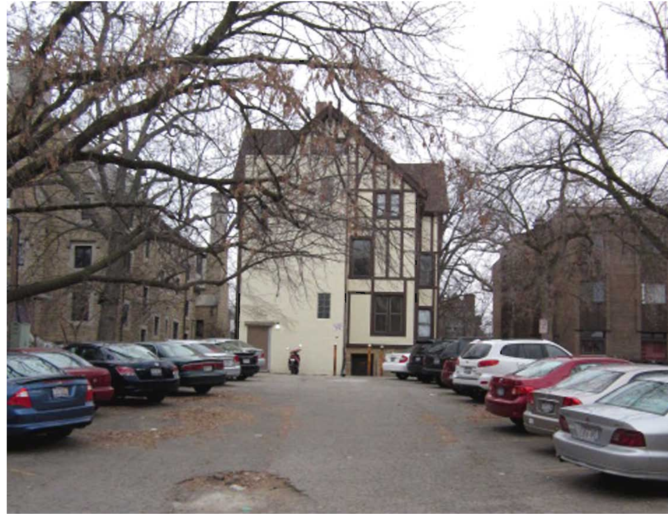
210 Langdon Street - Rear Elevation
