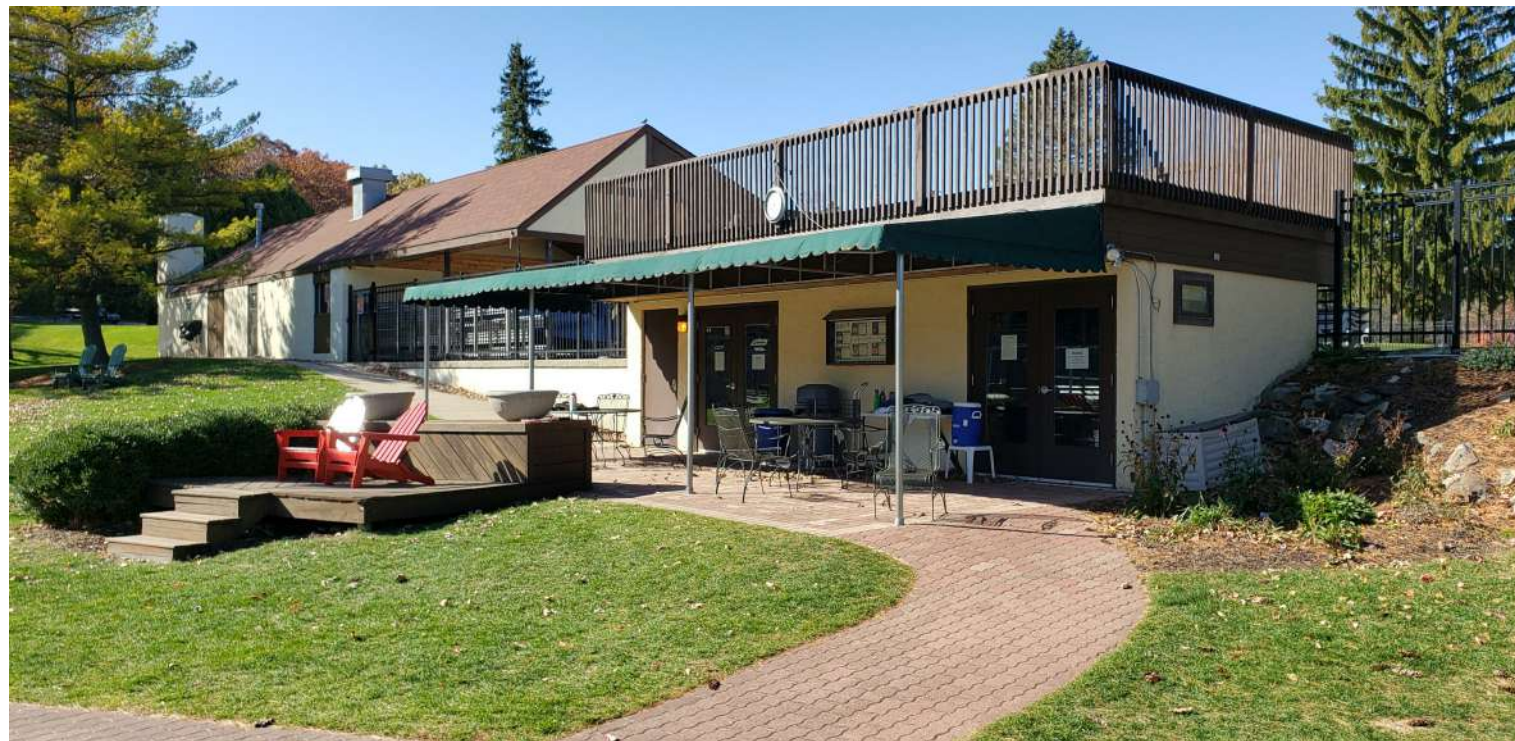
EXISTING EAST BUILDING FACE
