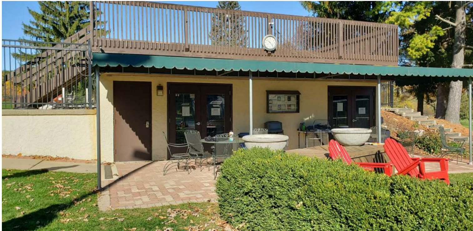
EXISTING PRO TENNIS SHOP
