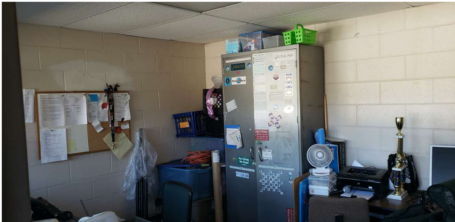
EXISTING LIFE GUARD OFFICE
