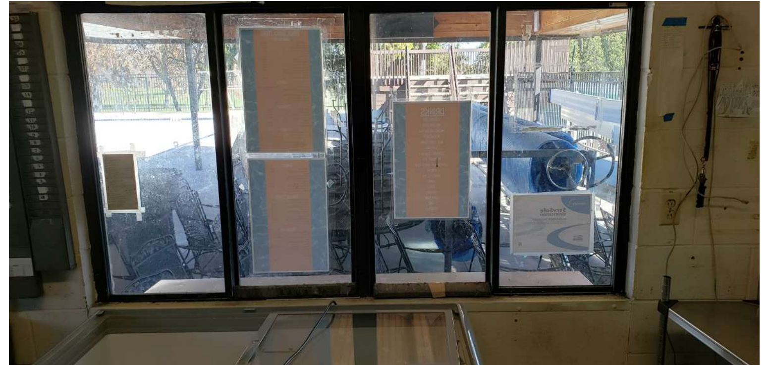
EXISTING FOOD SERVICE WINDOW
