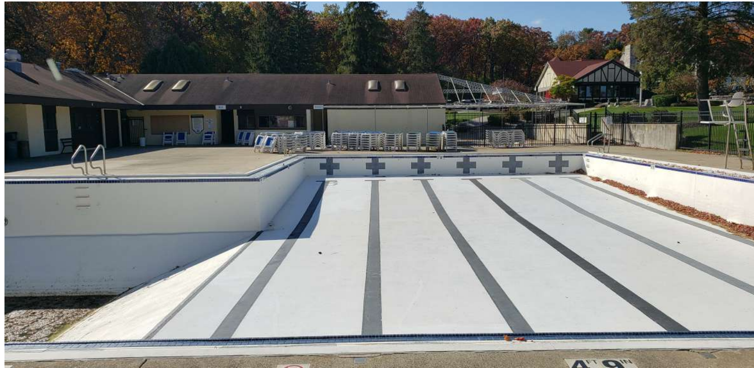
EXISTING NORTH BUILDING FACE
