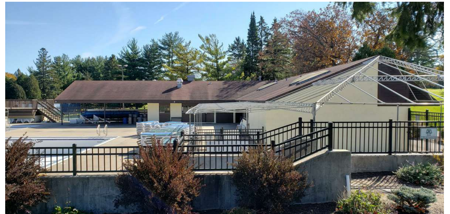
EXISTING WEST BUILDING FACE
