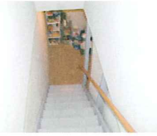
1105 Fish Hatchery Unit 2-3 Basement Stair.jpg
