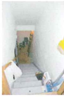
1105 Fish Hatchery Unit 1-4 Basement Stair.jpg
