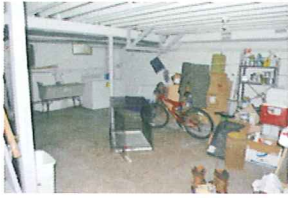
1105 Fish Hatchery Unit 1-4 Basement 1.jpg
