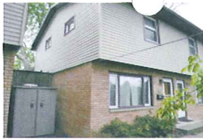
1105 Fish Hatchery Between Bldg View.jpg
