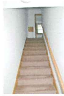
1105 Fish Hatchery Unit 1-4 Upper Stair.jpg
