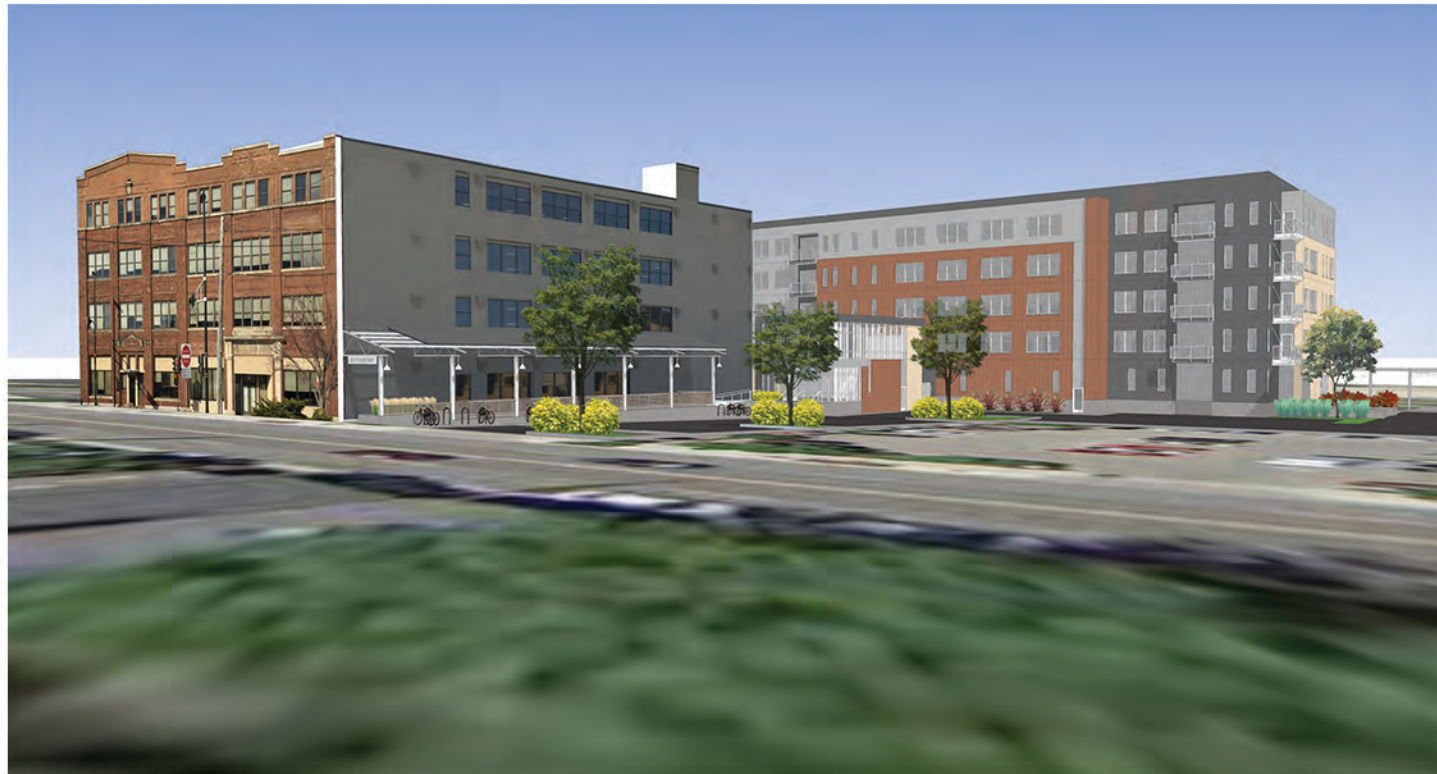
View from Williamson Street
