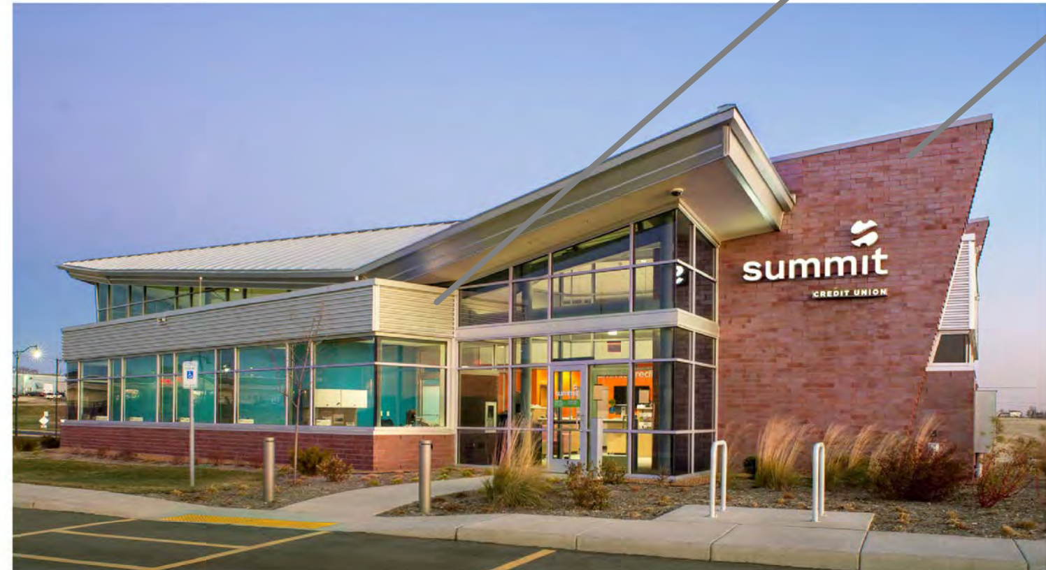
BRANCH WILL USE SAME RED BRICK AND RIBBED CONCEALED FASTENER RIBBED METAL PANELS AS MT. HOREB BRANCH (PICTURED)
