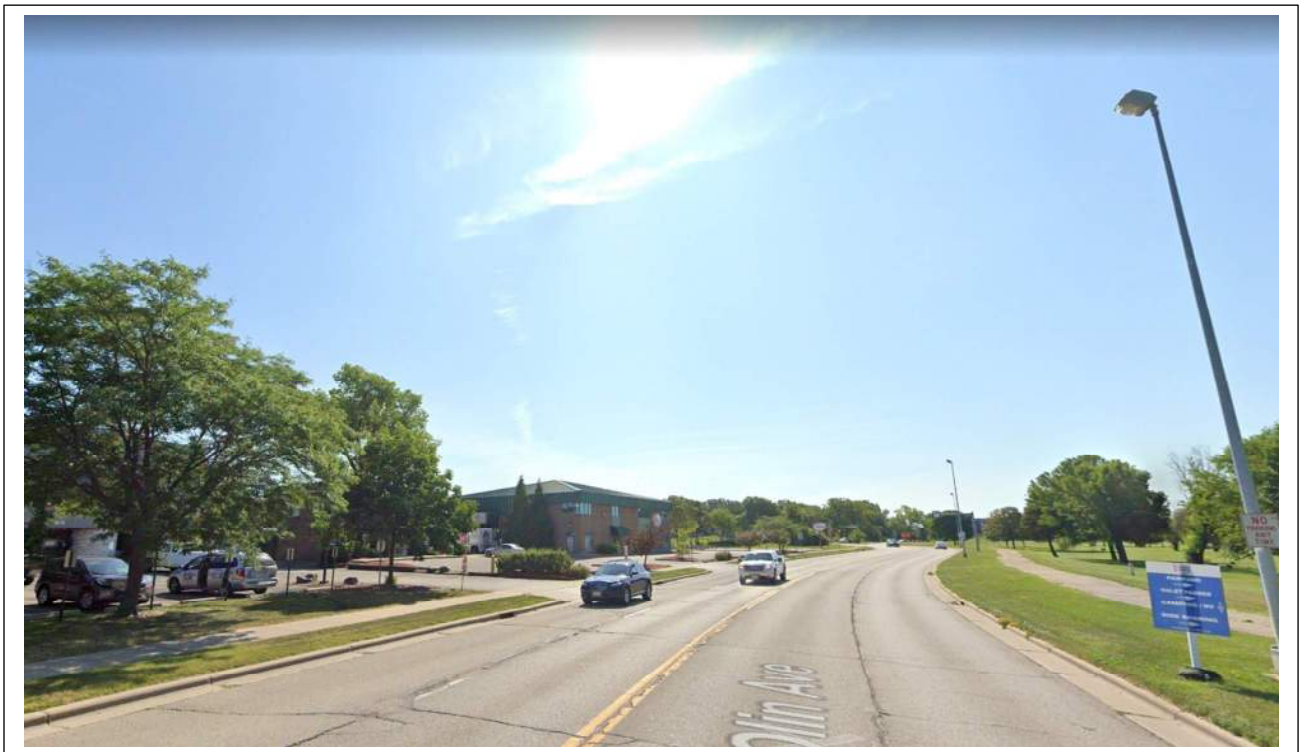
E. Olin Avenue – Facing East
