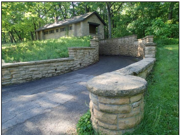
During the Great Depression, the Works Progress Administration and Civil Works Administration built stone entrances, the shelter, and fireplaces at Hoyt Park.
