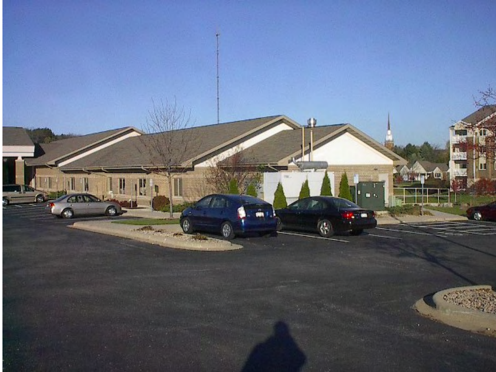
East end of Sebring Assisted-Care Residence
