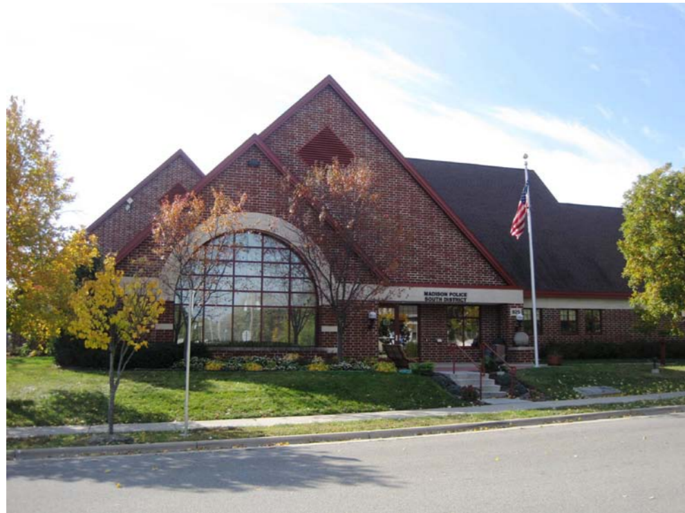
Police station to the west of the property.
