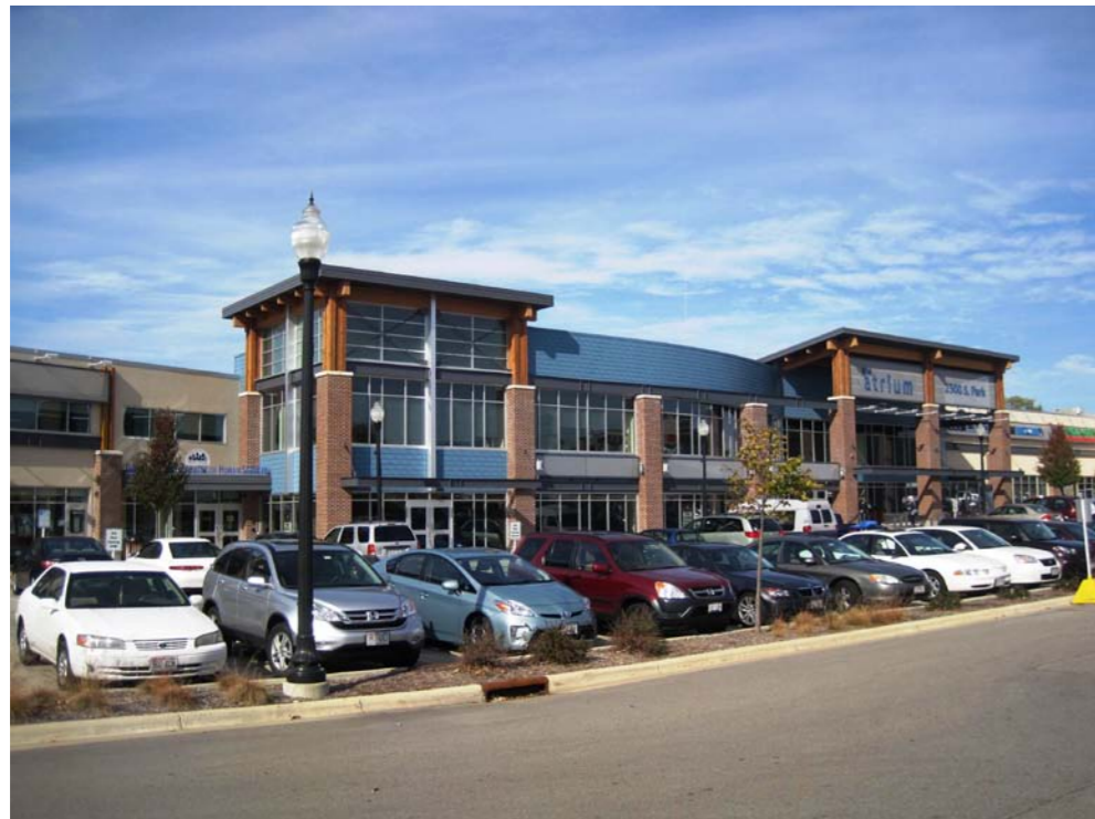
Atrium Building to the north of the property.
